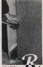
One method is to stiffen with plywood. Cover whole lower half of garage door and fasten with four-penny nails
