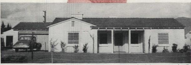
A stabilized earth house can be built anywhere if proper proportions of sand and clay are present in soil
