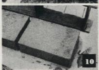
Blocks should not be moved until two days after form is removed to allow for hardening
