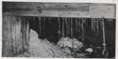
Moisture is essential to termite life. Stalagmitelike tunnels connect underground termite colony in earth with structural members of house
