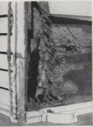
Damage to wood siding. Partly excavated or unexcavated soil area beneath ground floor is danger spot
