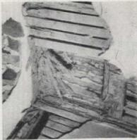
Termite damage to this interior wall was discovered only after outer wall covering was removed
