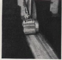
To start, No. 2½ sandpaper was used. Varnish, some paints require coarser starting paper. If floor is warped, go over diagonally in both directions, sand with grain. Next, buff floor with No. ½ paper. Fine floors require 3 or 4 sandings
