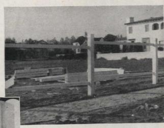
The fence shown here in stages was built in Los Angeles, Calif. in 1937-350 ft. of it, for about \$1.00 per ft. Specifications are
