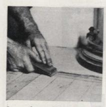
Remove floor mold and edger will finish to within ½ inch of wall. Countersink any surface nails, otherwise sandpaper will be ripped. Use handscraper around hearth. To resharpen scraper, use file. Always scrape in direction of the grain
