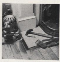
When first half of floor had been sanded, oil stain was applied (see types of finishes below). Pine, beech, maple and fir do not require filler, may be varnished or shellacked. Oak floors require filler, finished with sealers instead of varnish or shellac
