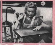
An aid to scraping off old paint-don't hold too close to the wood. Hold a few feet away to dry new paint
