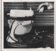
since these agents cut grease; then put a tablespoonful of new grease in the box. Be careful, also, to use grease of the proper consistency. It is necessary to grease about once a year, but if the mixer is in constant use, gears should be greased more frequently. See photograph above.
