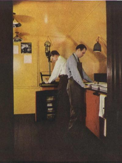
Proper working order from left to right leads from enlarger to trays for developer, shortstop and fix, and ends at sink
