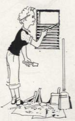
Chip away all plaster in opening, saw off lath at even flush with studs. Use keyhole saw or a hack-saw blade
