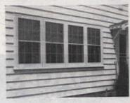
Hereisa corner installation of Curtis Silentite casements. These casements have no exterior hardware and are operated by a new method They cannot rattle or swing in the wind and are "insulated" to save fuel.
