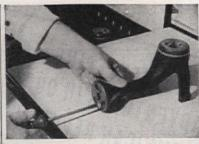
Loosen air shutter with screwdriver and turn up or down to control admixture of gas with air
