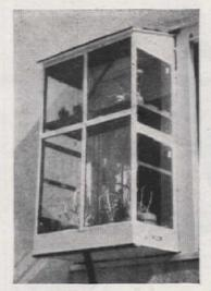
Five large screw-eyes on each side and a brace extending down to the cellar window frame hold Mr. Bullard's "conservatory " snugly against a weather strip
