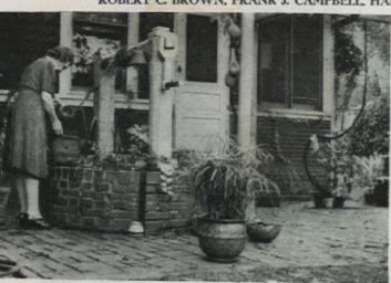
With the old pump removed and a 20" brick wall built around it, the cistern in the Proctor yard retained its usefulness, but became a colorful feature of the brick-paved, plant-decked terrace
