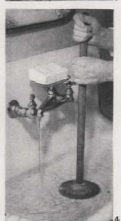
Plumbing pointers: 1. Label all shut-off valves: 2. Patch pipe temporarily with hinged, bolted iron clamp: 3. Remove plug at base of trap to get at obstruc-tion if use of rubber plunger (4) in sink doesn't do the job
