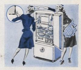
When all of the frost is gone, empty defrosting tray, clean freezer with solution of baking soda and water which helps get rid of food odors—leaves it "sweet." Then refill ice trays with fresh water and start the refrigerator.
