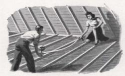
1. If your attic is unfloored, install Kimsul there. To determine quantity of insulation needed, measure space between two joists to get width of blanket required. Then multiply attic width by its length to get total square feet of insulation needed. If attic is floored install Kimsul in sloping roof. Remember to take measurements to your dealer.
