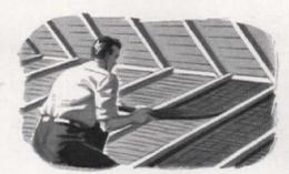
4. To install Kimsul in unfloored attic, use one of the many cleats that come with each roll of Kimsul to fasten one end of the blanket at junction of floor and eave. Pull blanket across attic floor, stretching it taut, and fasten to opposite eave. Repeat for each open section of floor. That's all!
