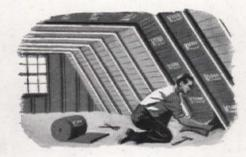
5. If your attic is floored, insulate attic roof instead. Cut lengths of blanket long enough to reach from eave up to collar beam, across beam and down roof to the opposite eave. Use the cleats to fasten KIMSUL in place as you go. An attic roof is easy to insulate with KIMSUL! See illustration above.
