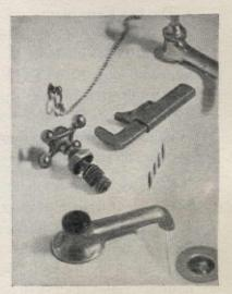
Unscrew cap until it is free, then unscrew and lift out valve stem with the critical washer at its end
