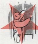
FLEXIBLE insulation is perhaps the most commonly used type in home construction. Its loose density makes it ideal as a heat retardant. Usually placed between studs, joists or rafters, it is extremely light in weight and very easily installed. Today, most flexible insulation comes in the form of batts or in blankets covered on either one or two sides with moisture resistant paper. This vaporseal paper
