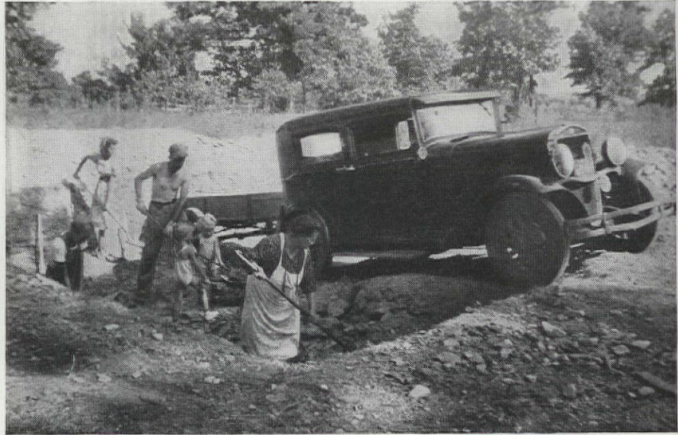
Teamwork is the slogan of the six Swansons of Seneca, Illinois
