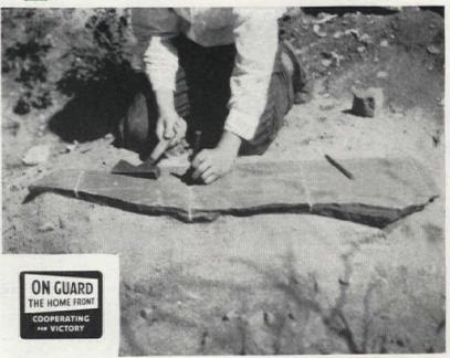
To cut stone, lay it flat on sand; chisel all way around, gradually increasing weight of blows. Use scraps for wall and steps
