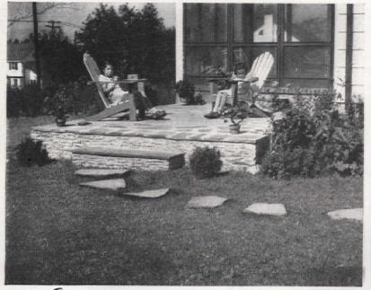
6 For neat, trim effect, keep the stone surfaces clean of cement and remove surplus from joints while it is soft
