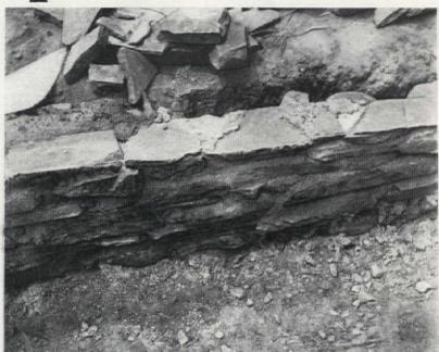
Ten-inch walls on a foot or more of concrete footing are faced with cemented flags, then filled with stones and mortar
