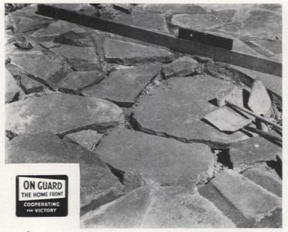
4 Use straightedge and level to avoid low spots, puddles, and frost cracks. Bed stones firmly in soft, rather wet cement
