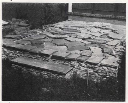
5 Shape and fit surface stones before cementing. Height of broken stone base and flagging should be about eight inches
