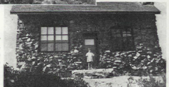
The front and rear views and, above, a close-up of the stone construction
