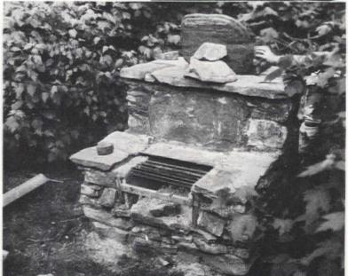
Figure 6. A wind shelf was built in to prevent back drafts
