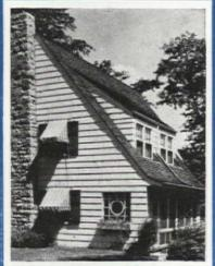
Double-walling with Cedar Shingles is very beautiful and very substantial. The shadow lines are deeper . . . the insulation much greater and the cost no more because the shingles are laid with a wider exposure to the weather, not practical by the old method of single-coursing.
