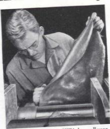
Our Own Rubber Mill is busy all year with samples and experimental batches. This sheet of pure rubber will be a new-type Plymouth body mounting.
