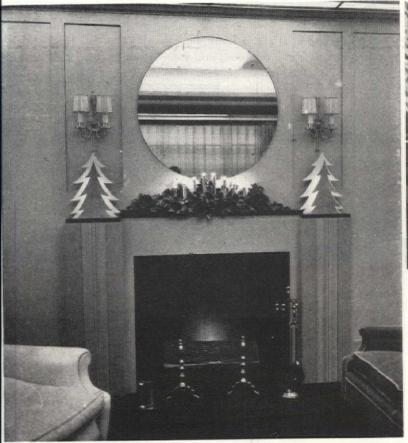
The flat trees are of multiple construction, each containing three lowwattage lamps concealed between the planes. The eight candles are operated in series on a single circuit. A very effective use of lights
