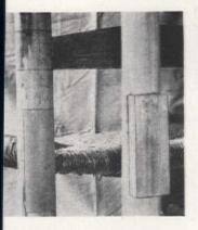
he leg at left was completely sheared off, he model at right shows how extra piece as set in. The extra wood was planed own and finished with a file and sandaper. When possible two of these pieces splints set opposite each other make a mains of the one-time gorgeous design was one faint gold line about 3% of an inch long. And the old swing-leg maple dropleaf table I carried away for \$2.75 was rapidly becoming decomposed. Such a table!
