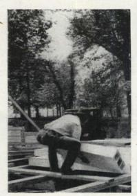
construction of Gypsum lumber a product of the Rockwood Corp. Above laying floor units for a new house
