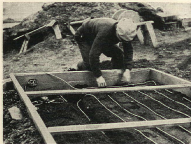
Another method is by installing a specially designed type of heating wire, lead covered, imbedded in the soil or even laid on the surface
