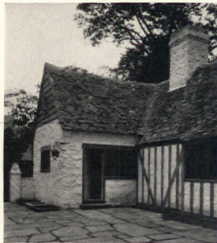
Flat terra cotta tiles in a wide range of reds complete the picture of this charmingly faithful reproduction of a typical French farm cottage. Frank Forster, architect. Courtesy, Ludowici-Celadon Co.
