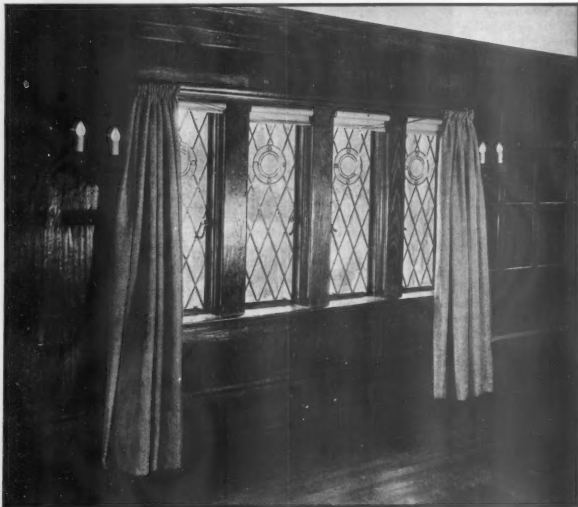
With the boiler type of heating plant one can use concealed radiation like that barely visible along the baseboard of the room at the left. Humidification sections are used with this kind of concealed radiation, as described in the text. (Courtesy, Bon-Air Corp.)
