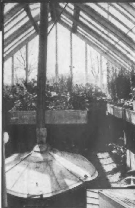
A greenhouse that is easily assembled and constructed, for the most part, of cold-frame and cellar window sash
