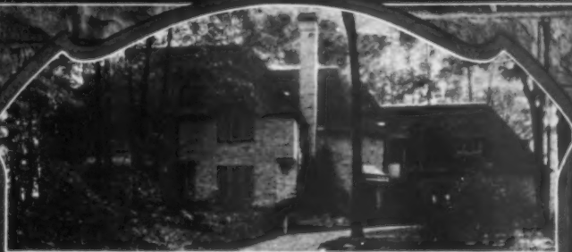
E. S. Warner Residence Shaker Heights, Ohio
