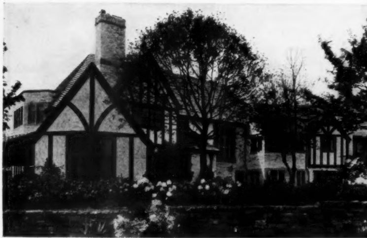
House in Portland, Ore., Kirtland Cutter, Architect. Cabot's Blended Roof Shakes; Cabot's Old Virginia White on brickwork. Cabot's Quilt in walls to deaden noise and make the house warm and livable.
