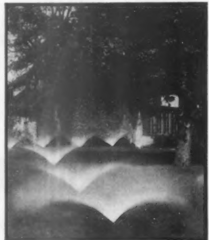
Sunk down to the grass surface when not in actual action, these outlets to a permanent modernized installation are for the perfect lawn
