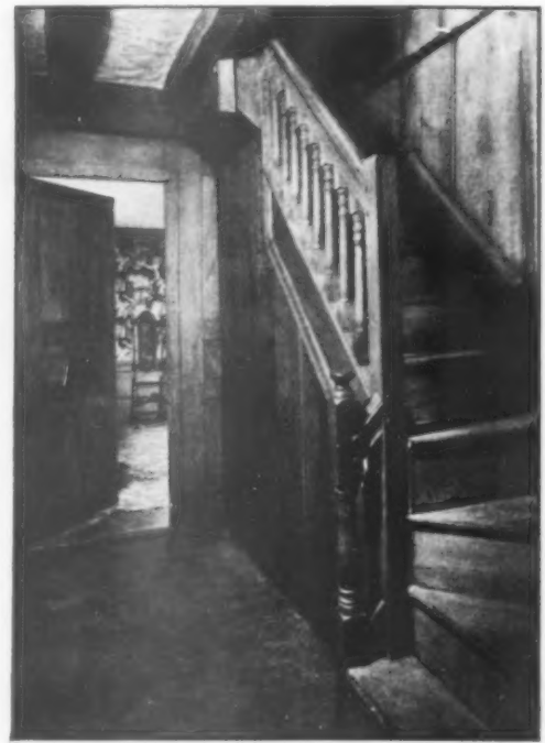
The hall and stairway in an old New England colonial house, showing panelled walls and beamed ceiling
