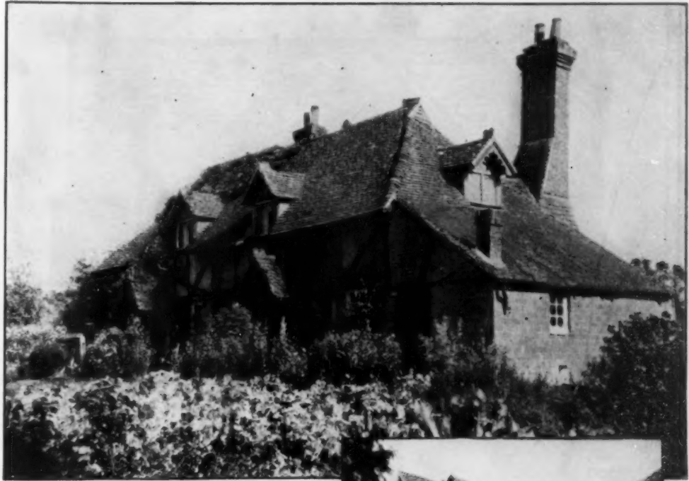
Like our own Dutch Colonial houses the buildings in Surrey make use of many materials. In the photograph above, we see stone, brick, and half timber lending each its individual charm to the wall
