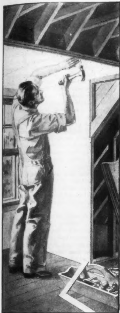
Stop the leakage of furnace heat by nailing Celotex to the underside of roof rafters. The big, strong boards add lasting strength to roof structures. You'll find them easy to apply just like lumber with hammer and large headed nails.
