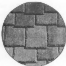
Picturing the Westminster the ched lay of Pennsylvania Blue-Grey Slate, butt cut dressed, smooth texture. (P. S. I. Spec. 31C)
