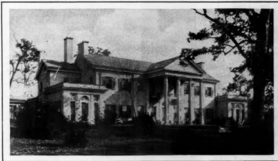
The Houston home has concrete masonry walls throughout, with white portland cement stucco exterior. Reinforced concrete floor above basement, which extends under a part of the home only.
