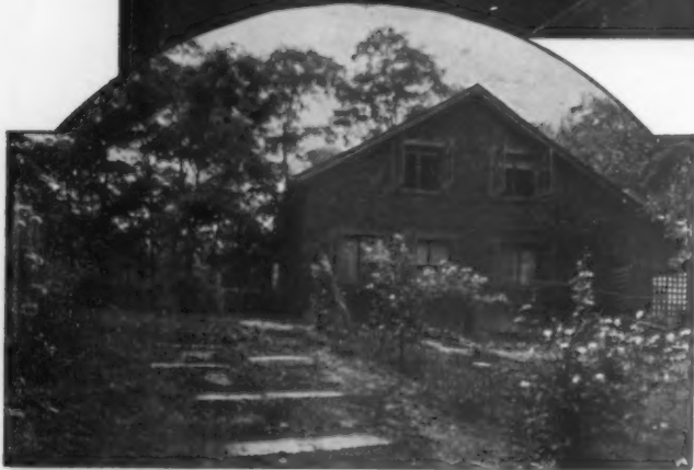
A flight of twelve wide stone steps leads up from the roadway, to where the little brown home stands with wide casement windows open to the four winds and all the sunshine there is
