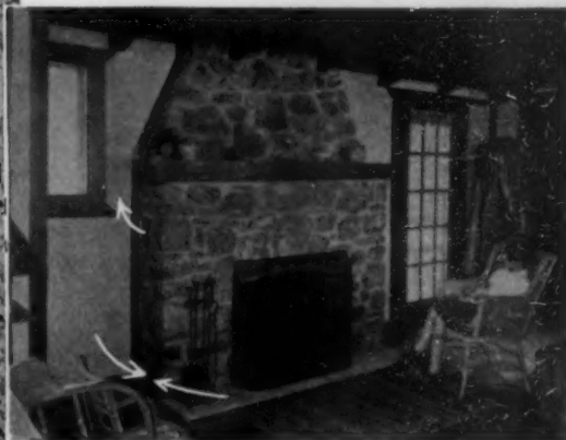
Arrows show circulation of air through the Heatilator grilles and heating chamber. This installation is at Sports, N. J. N. A. Hall, Owner, Edwin Closs, Architect.
