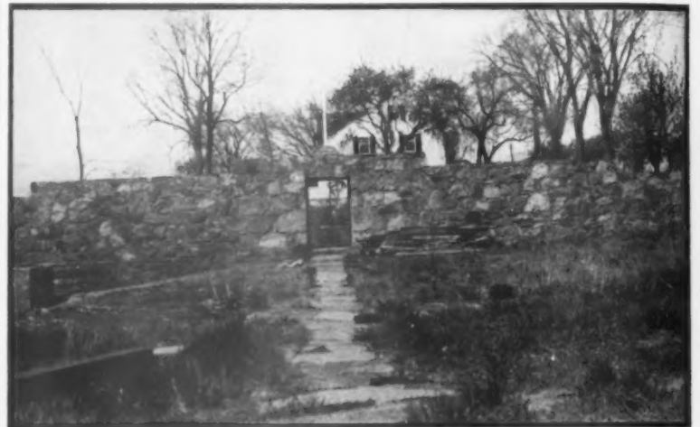
The garden wall and old wrought iron gate leading directly to Mr. Durant's door
