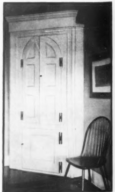
The original corner cupboard in the dining room: the old paneling and wrought iron hinges are most interesting
