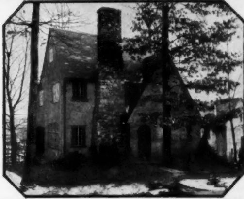
The finished dwelling, built of stucco, with a slate roof, at a total cost of $17,600—a price which includes the ground
