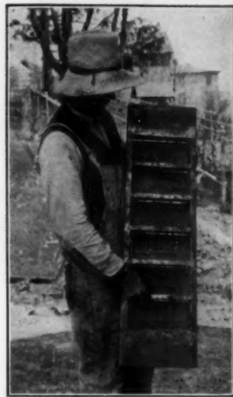
Here's one of the moulds that our Old Virginia Brick are made in. It's exactly like those Jefferson made his in.
