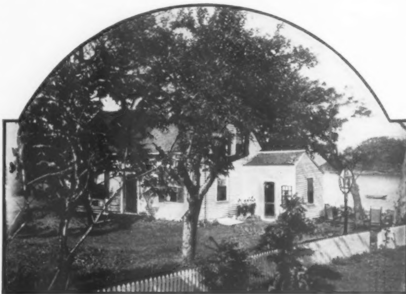
At Barnegat, Marblehead, Mass., stands this sturdy and simple New England house which a little remodeling has made into a comfortable dwelling
