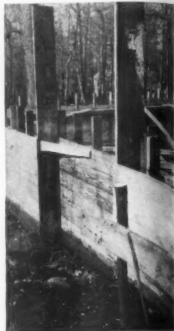
Inside form for concrete foundation
