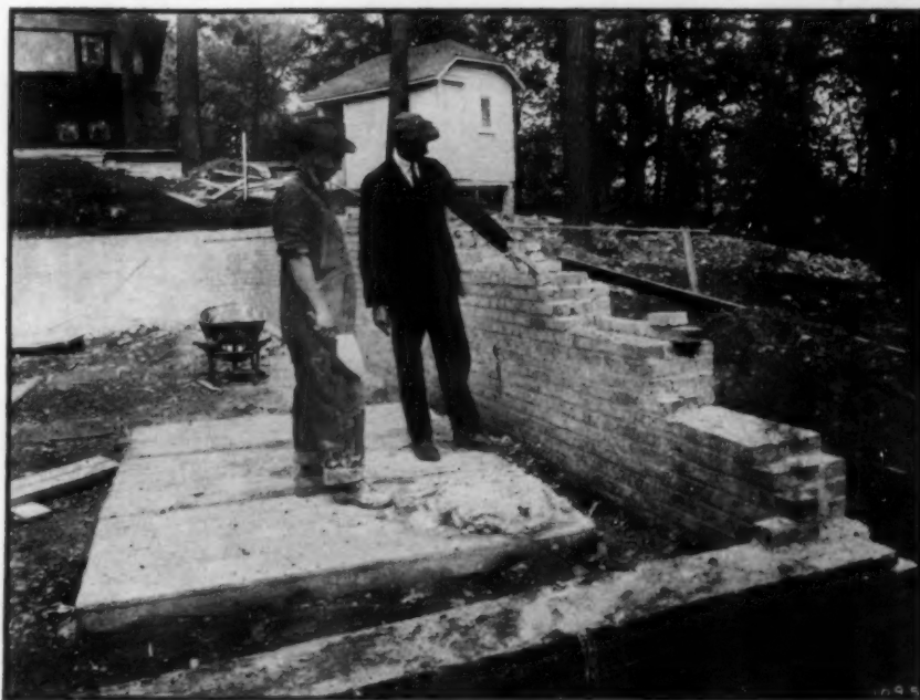
A brick foundation during construction
