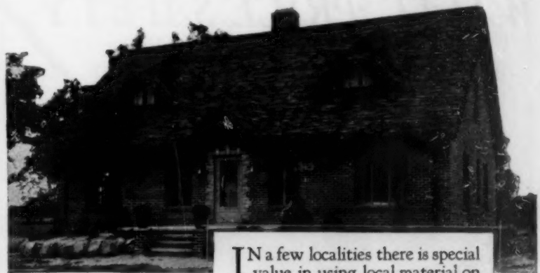
WEATHERBEST Roof in weathered straw colors, designed by owner Rule D. Egbert, Tiffin, Ohio.
