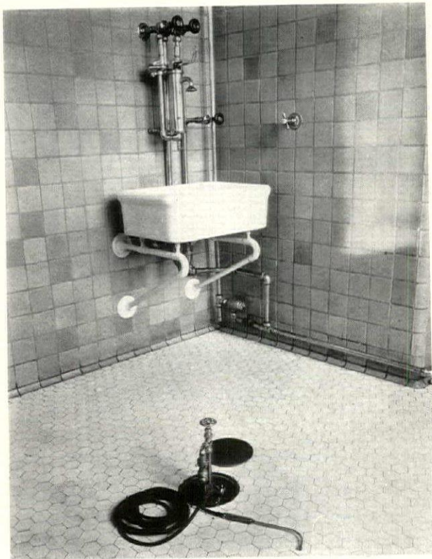
Figure 1 (left). Distilled water outlet in operating room with electric reheater; also showing aspirator attached to floor drain. Figure 2 (above). Another distilled water outlet for surgeons' scrub-up, with exposed reheater and elbow control
