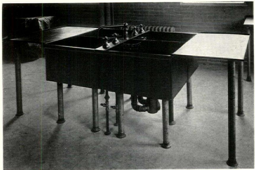
Figure 12. A four-part kitchen sink that stands free from walls and partitions so it may be easily cleaned inside and outside, equipped with swinging arm supply
