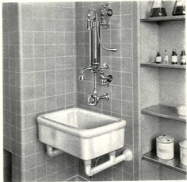
Figure 1 (left). Distilled water outlet in operating room with electric reheater; also showing aspirator attached to floor drain. Figure 2 (above). Another distilled water outlet for surgeons' scrub-up, with exposed reheater and elbow control
