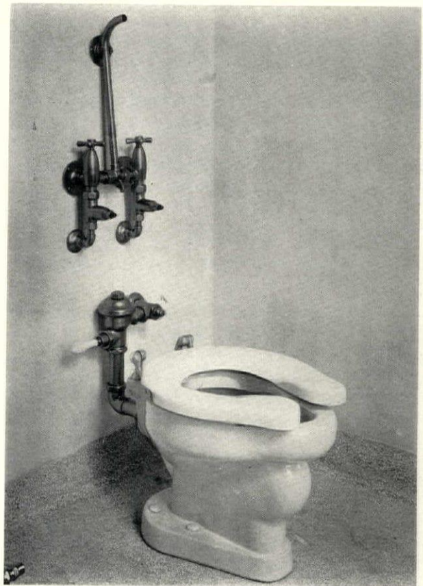
Figure 4. China water closet, with extended lip, Crescent seat, flushometer, and bed pan washing device on the wall
