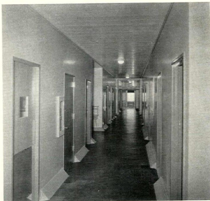
Hospital hardware consisting of adjustable friction hinges, a soft rubber roller in place of the usual noisy latch, an arm hook in place of a knob, and a sound absorbing ceiling, such as that shown at the right, are efficient for muffling noise in corridors
