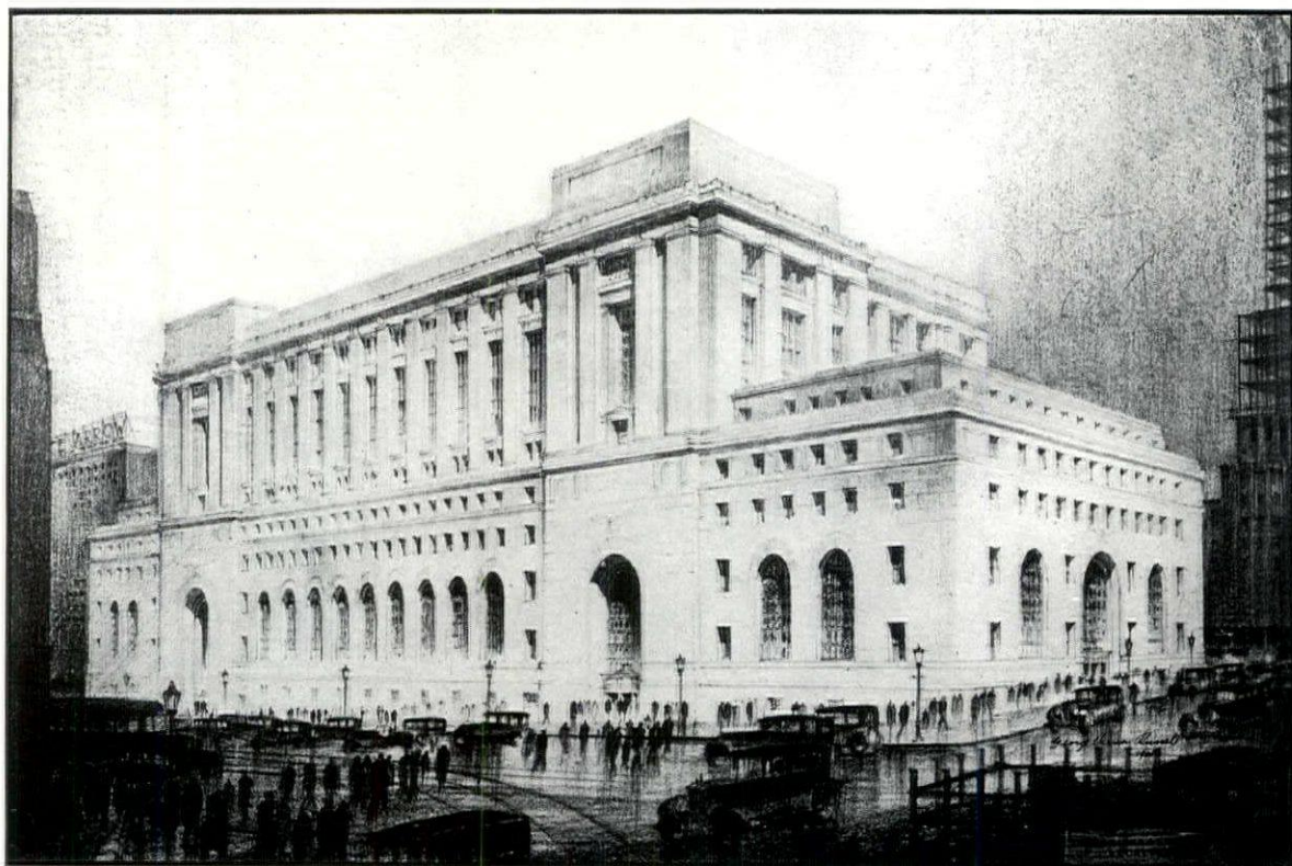
POST OFFICE AND COURT HOUSE PITTSBURGH, PA. TROWBRIDGE & LIVINGSTON, ARCHITECTS
