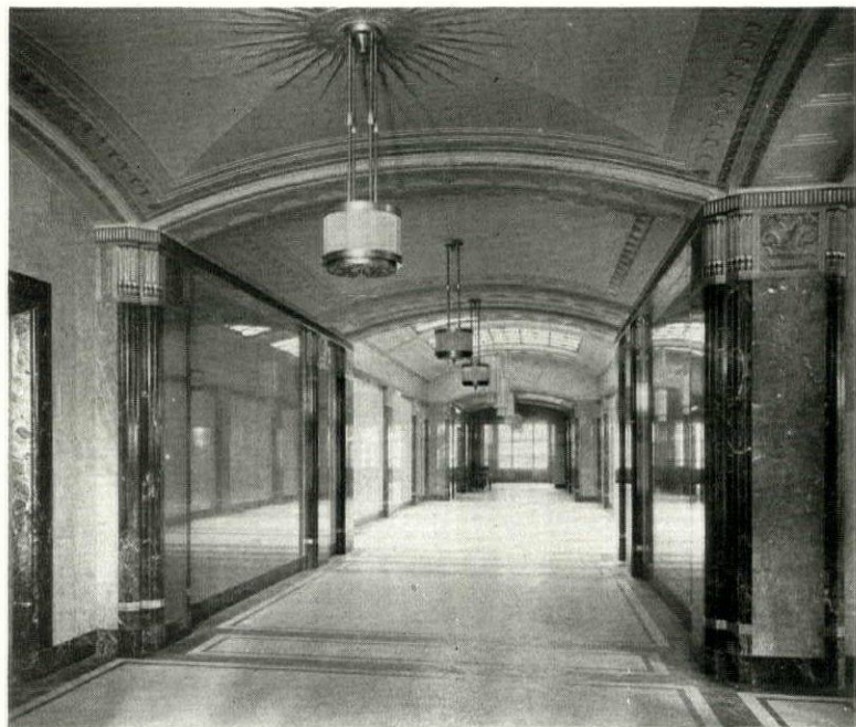
FIRST FLOOR CORRIDOR
