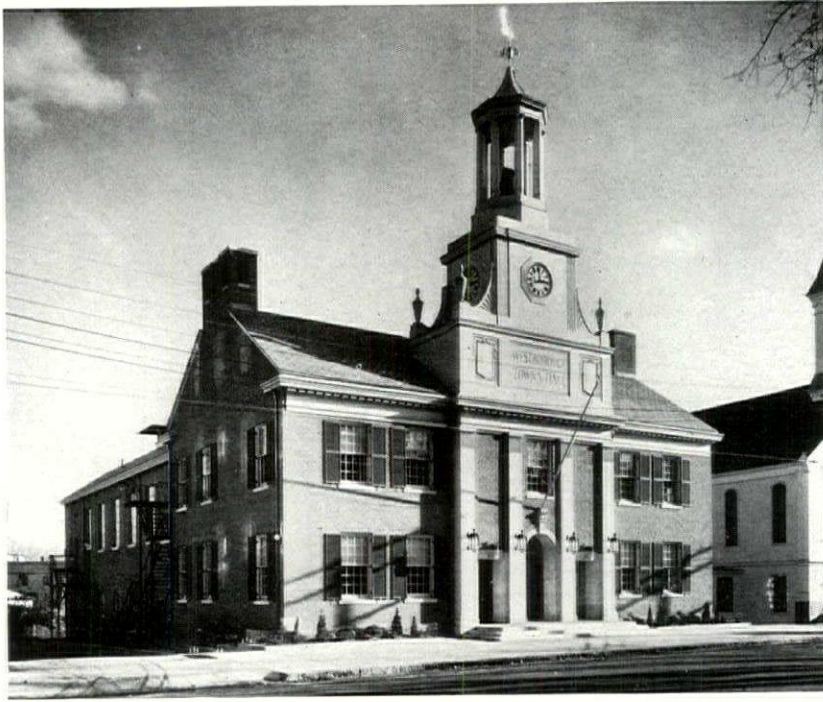
Town Hall, Westborough, Mass., is a modern adaptation of the Colonial, appropriate to an old and long settled community
