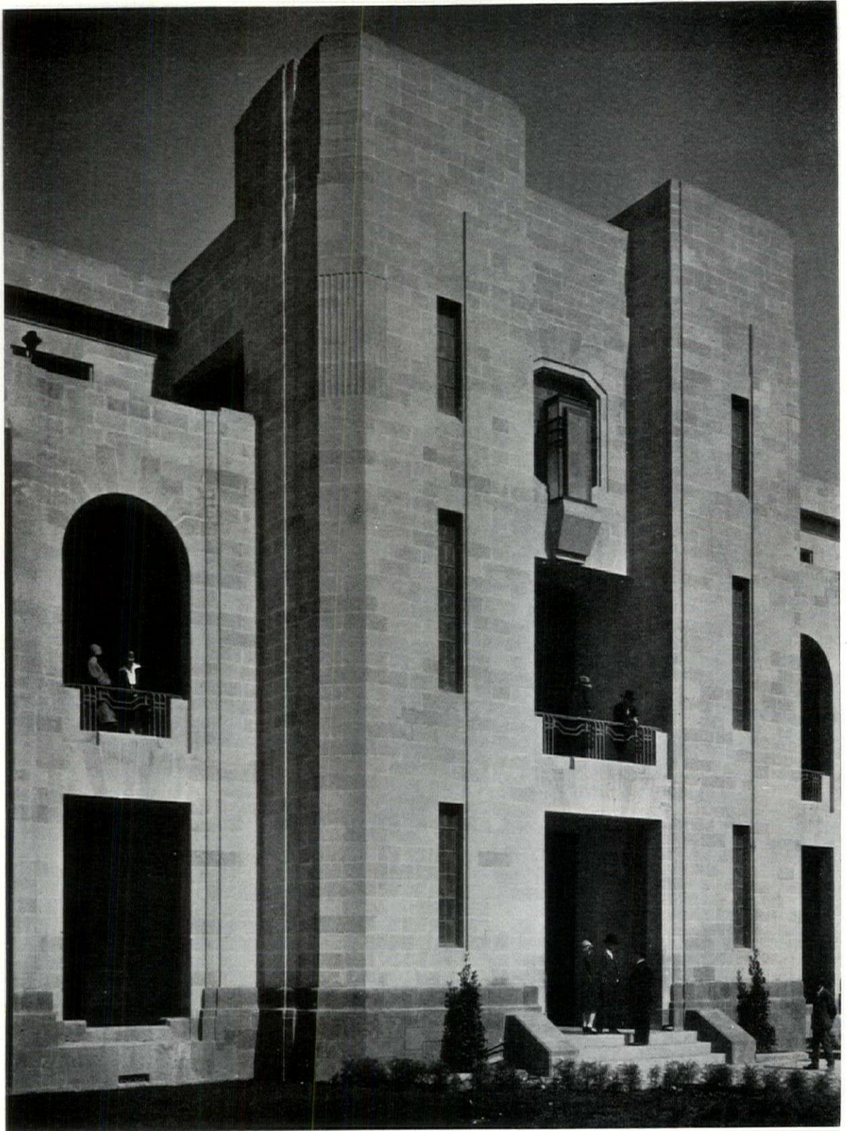
ENTRANCE TO THE MAIN BUILDING FROM THE PATIO
