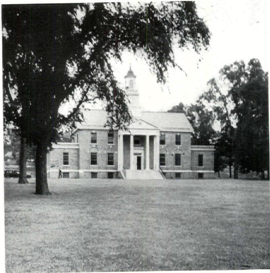
The municipal building at Teaneck, New Jersey, another small community which has realized the importance of maintaining a civic center of sufficient size to allow of growth without constriction
