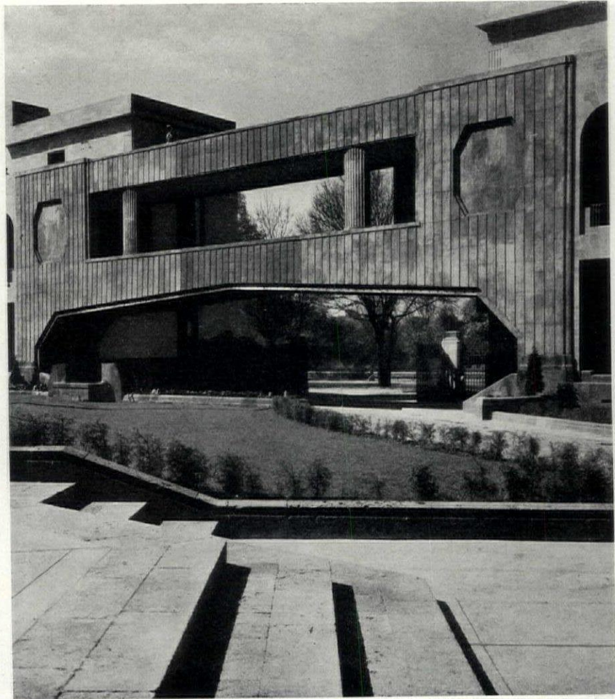
One of the bridges over the two main entrances into the patio. Notice the unusual form of the arch to express a truss form in stone and the simple vertical treatment of the bridge wall surface
