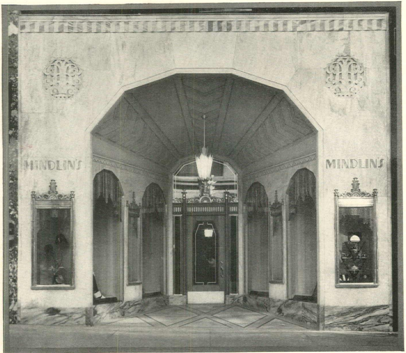
"MINDLIN'S," KANSAS CITY, PINK GEORGIA MARBLE Greenbaum, Hardy & Schumacher, Kansas City, Architects
