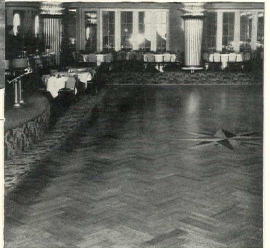
Pavilion Caprice (Night Club); dance floor in mastic blocks of quarter-sawn white oak, herringbone pattern. Note star motif in center panel reproduced in satinwood and teak.
