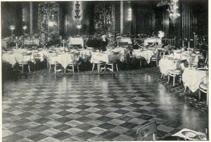
Main Dining Room with dance floor of clear American walnut mastic squares laid diagonally.
