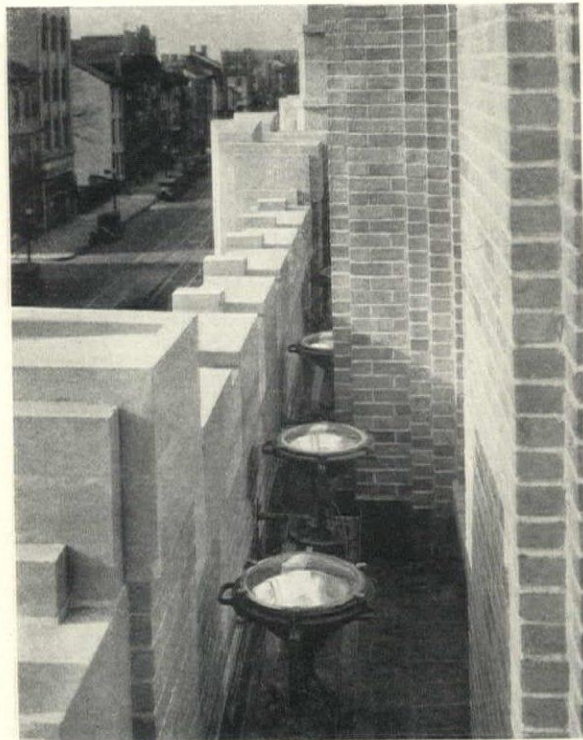
Location of projectors on a narrow setback of the Pennsylvania Power and Light Co. Building
