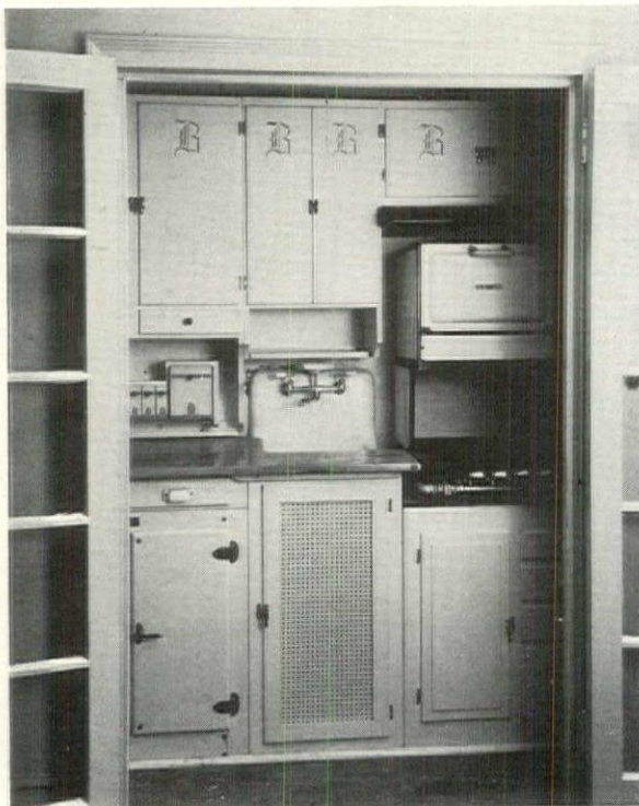
A Poor Arrangement. Unit Doors Swing in Wrong Directions; Sink and Drain Installation Is Unsanitary and Difficult to Keep Clean, and Counter Space Is Inadequate. Units Are Cramped Behind Doors
