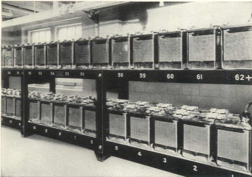
HERE IS AUTOMATIC PROTECTION FOR LIGHTS, POWER. Picture shows a typical Exide Emergency Lighting Battery in glass jars, which make inspection easy. The cells are arranged in neat, compact racks and are placed in the basement of buildings near the engine room. They take up little space and can readily be kept spotless and clean.
