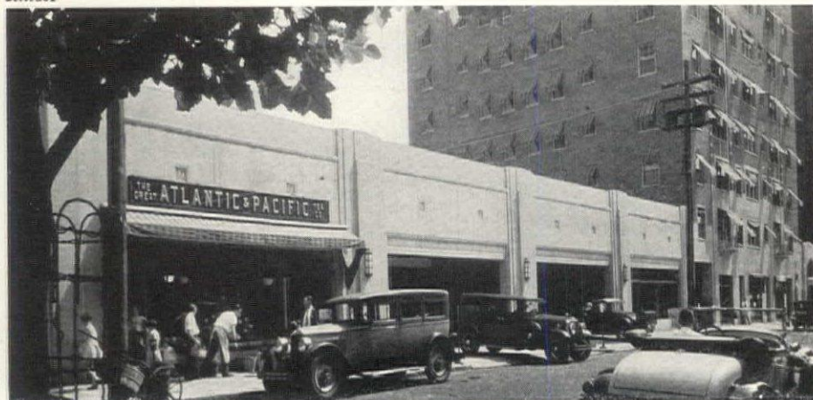
Entrance to Garden Court Garage
