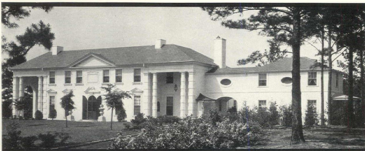
Thirteen telephone outlets, including one in the servants' quarters over the garage, provide for complete telephone convenience in the home of Dr. LeRoy Childs, Tuxedo Road, Atlanta, Georgia. Conduit for the telephone wiring is built into the walls and floors. HENTZ, ADLER & SCHUTZ, Architects, Atlanta.
