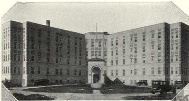
Little Company of Mary Hospital, Chicago, which has a laundry installed with the co-operation of American Laundry Machinery Company engineers.
