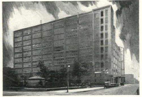
Duriron carries the acid wastes in Central Motor Repair Bldg., Dept. Plant & Structures—New York City Wells & Newton Co., Plumbing Contractors
