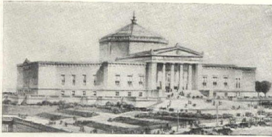
John G. Shedd Aquarium of the Field Museum, Chicago. Architects—Graham, Anderson, Probst & White. Plumbing Contractor—R. J. Powers
