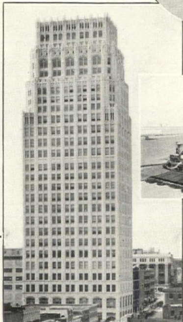
Below—2" Armstrong's Corkboard insulates the N. Y. Telephone Building, Buffalo. Architect—Vorhees, Genelin & Walker.
