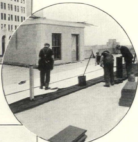
Below—2" Armstrong's Corkboard insulates the N. Y. Telephone Building, Buffalo. Architect—Vorhees, Genelin & Walker.
