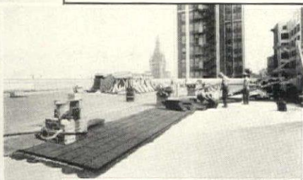
Below—2" Armstrong's Corkboard insulates the N. Y. Telephone Building, Buffalo. Architect—Vorhees, Genelin & Walker.
