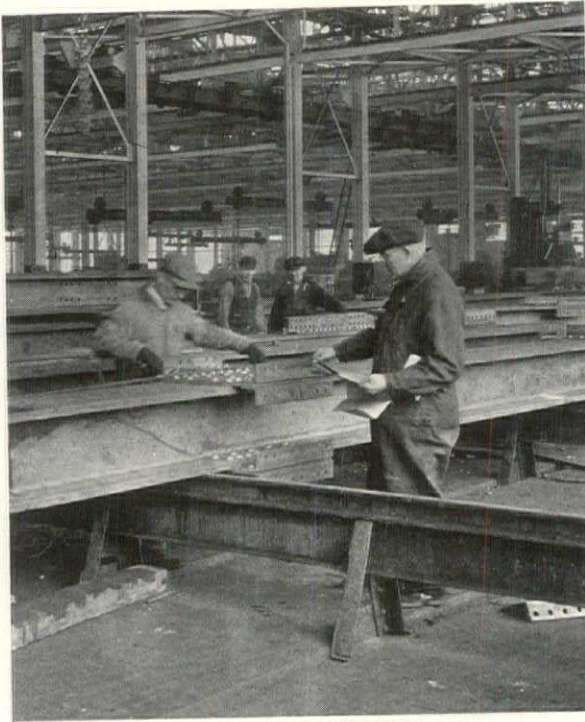
Shop inspection of fabricated steel saves delays
