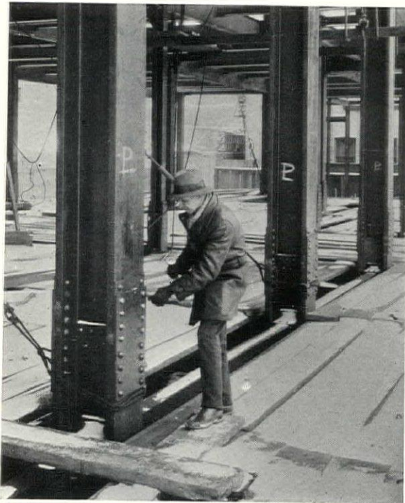
Testing rivets for tightness is part of the field inspection
