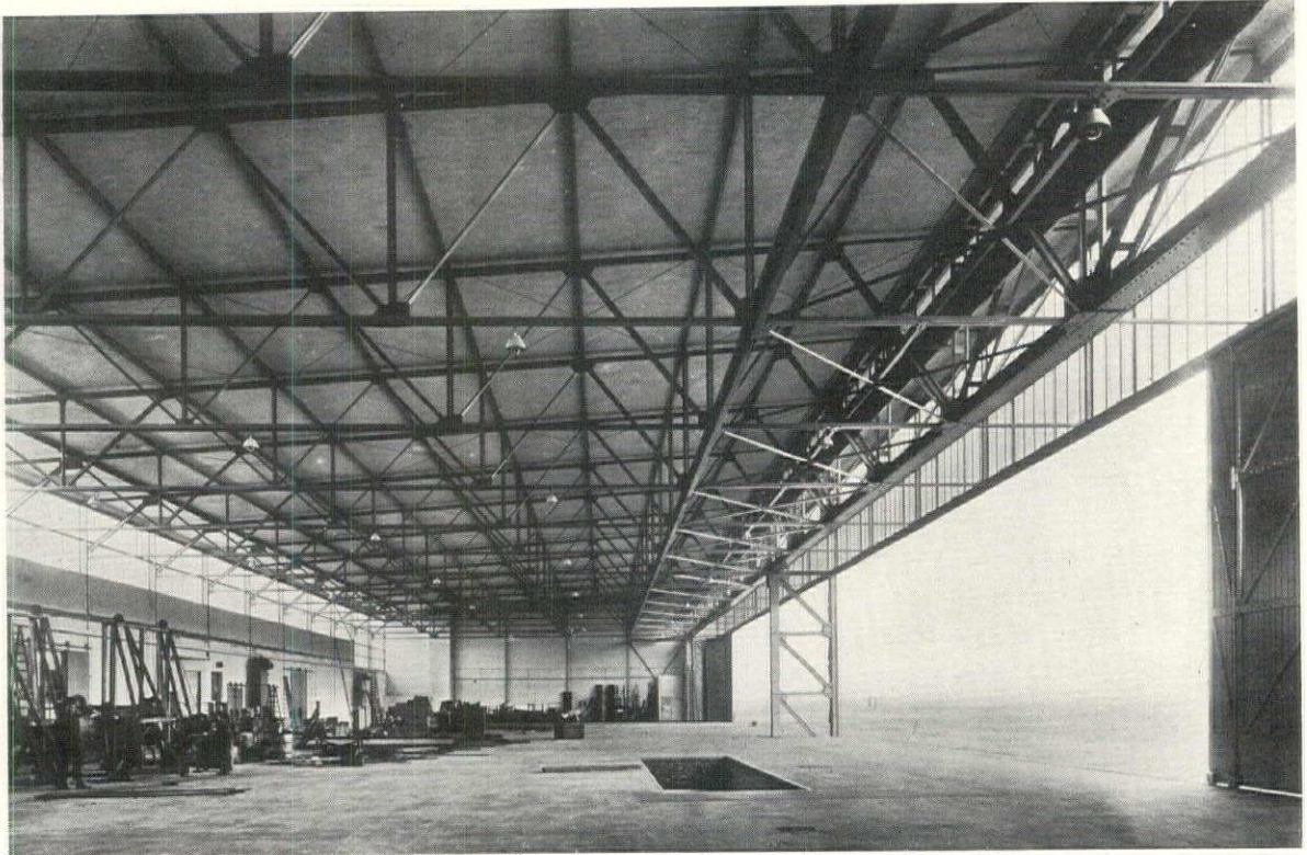
Interior of Tempelhof Hangar with Doors Open
