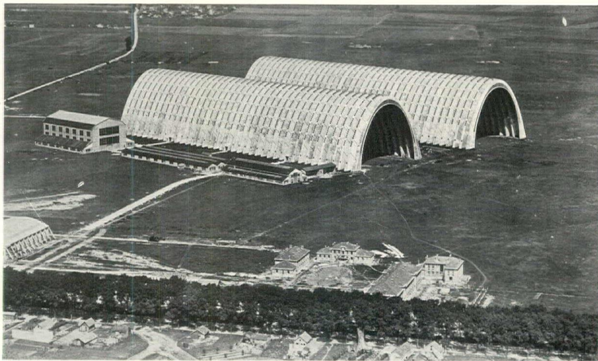
The Reinforced Concrete Hangars at Orly, near Paris
