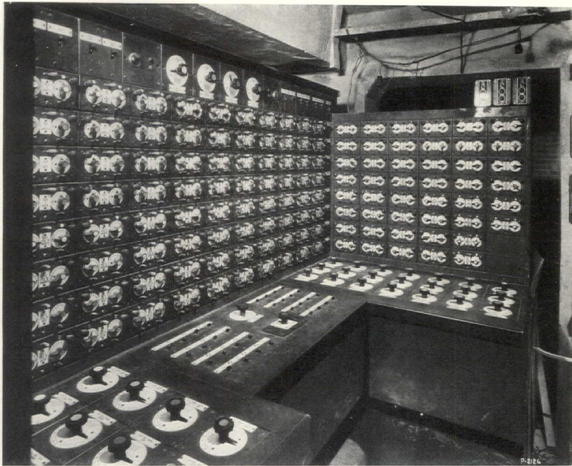
The Main Stage Lighting Control Board, Occupying a Position Next to the Prompter's Box
