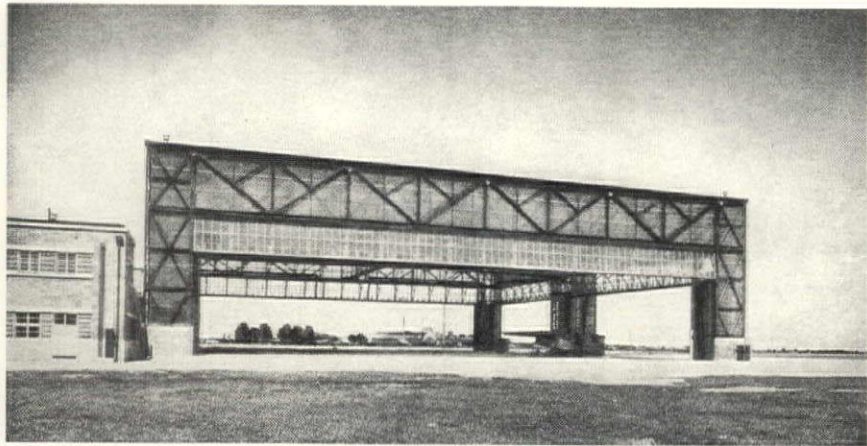
The Munich - Oberwiesenfeld Airport Hangar with all of the Doors Open on Three Sides of the Structure
