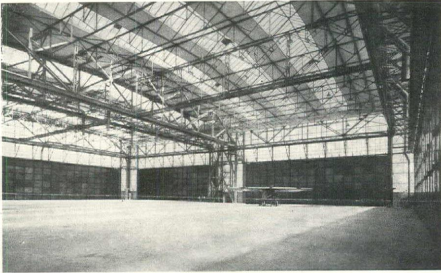
Interior of the Munich-Oberwiesenfeld Hangar Showing Interior Daylighting with the Doors Closed
