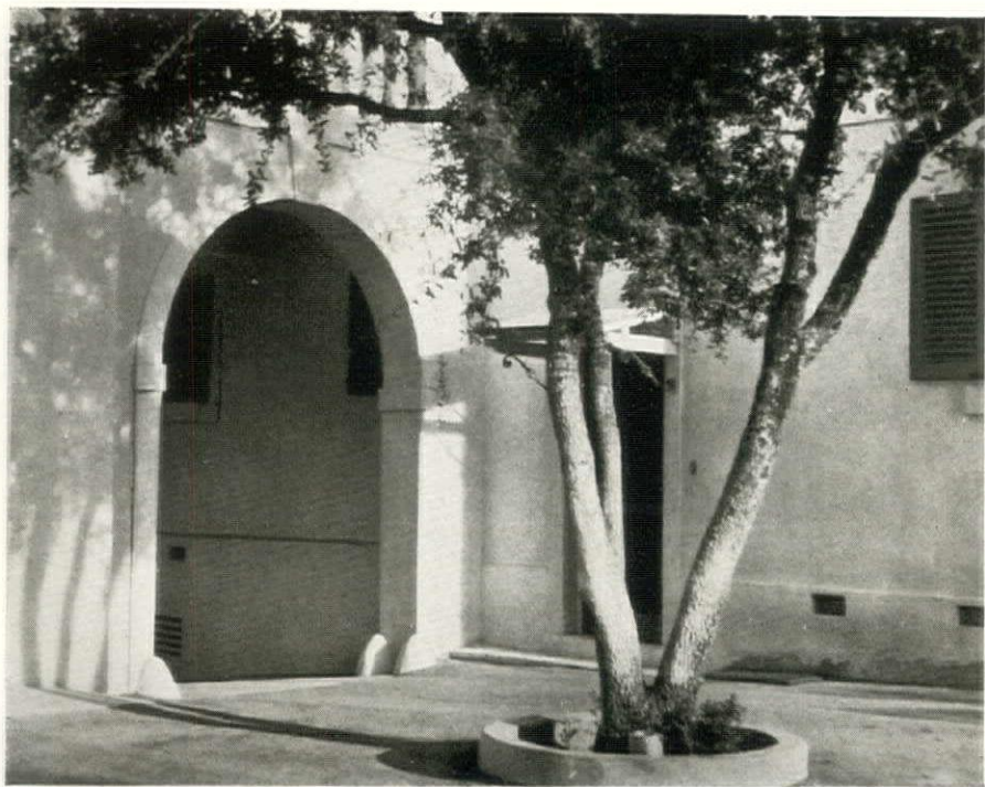
DRIVEWAY ARCH, SIDE DOOR AND REAR COURTYARD WITH OLD TREE
