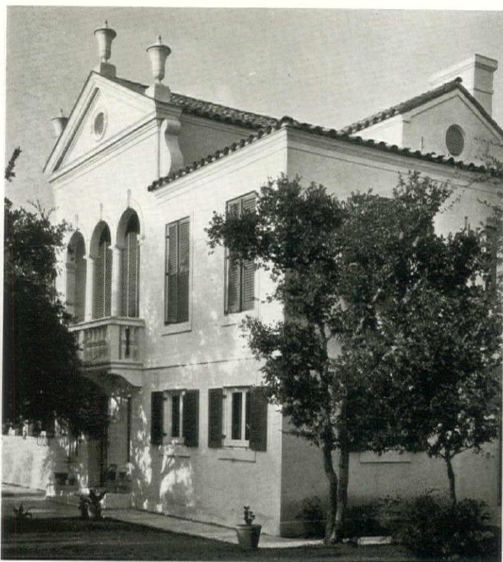
HOUSE FOR J. B. ROBERTSON, ESQ., AT SAN ANTONIO. WILLIAM McKNIGHT BOWMAN, ARCHITECT
