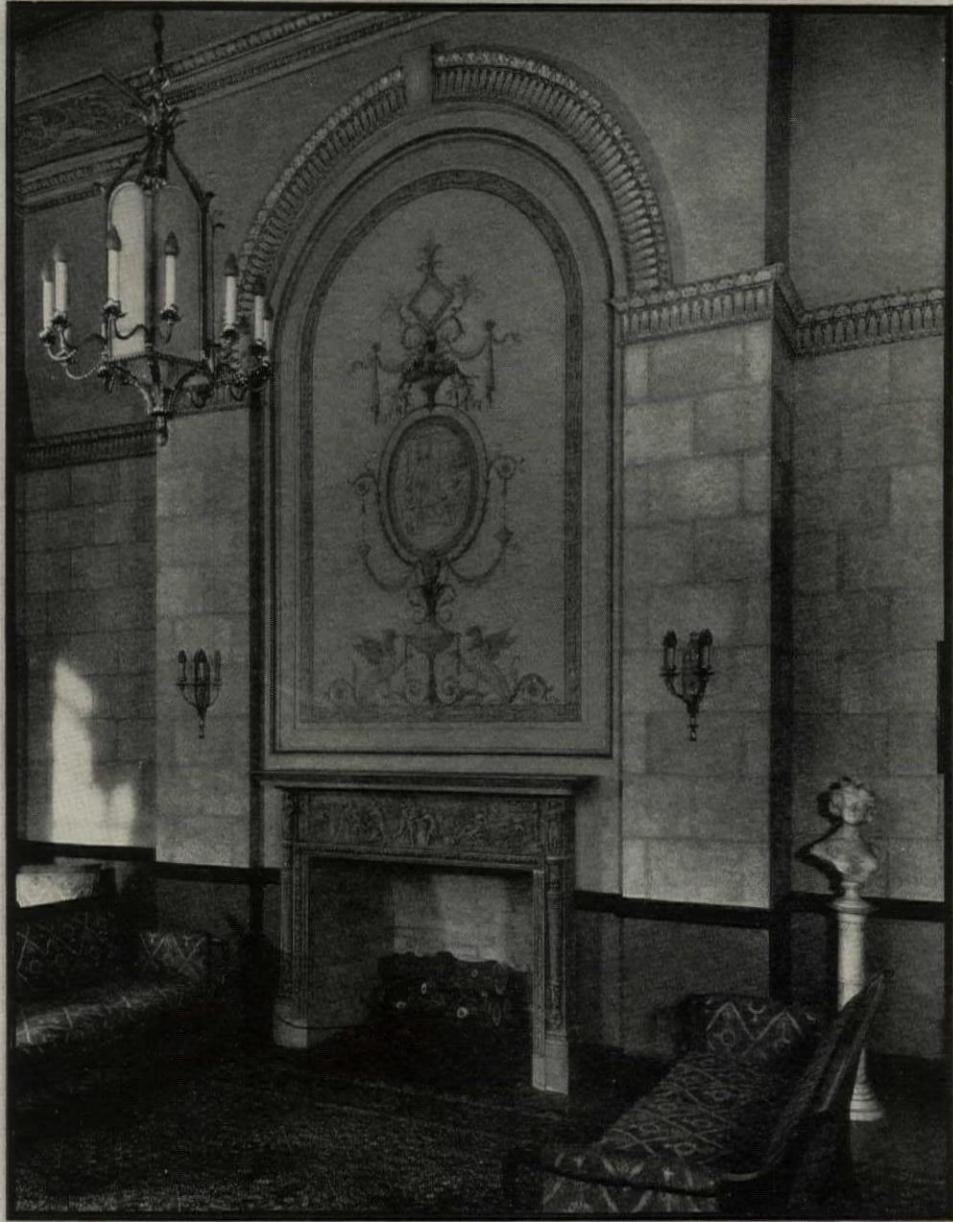
Zenitherm Wall in reception room, Stark County Tuberculosis Hospital, Louisville, Ohio. Albert L. Thayer, Architect
