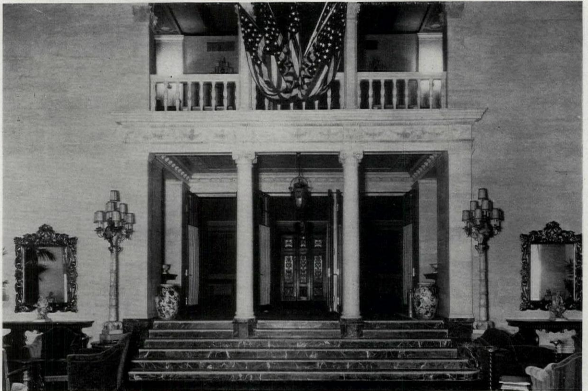
ENTRANCE TO BALL ROOM FOYER HOTEL STATLER, BUFFALO GEORGE B. POST & SONS, ARCHITECTS
