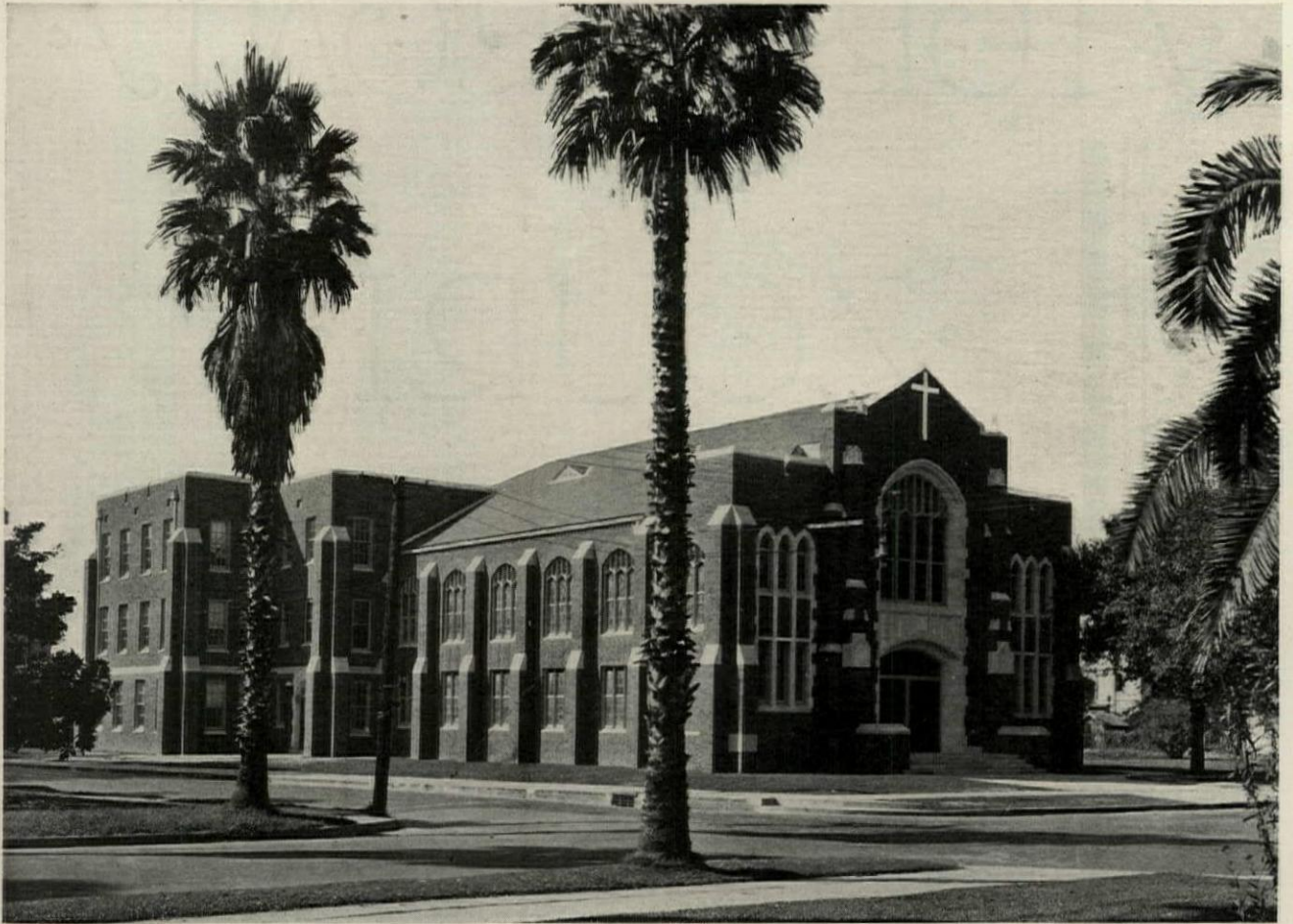
BROAD STREET METHODIST CHURCH, LAKE CHARLES, LA.
