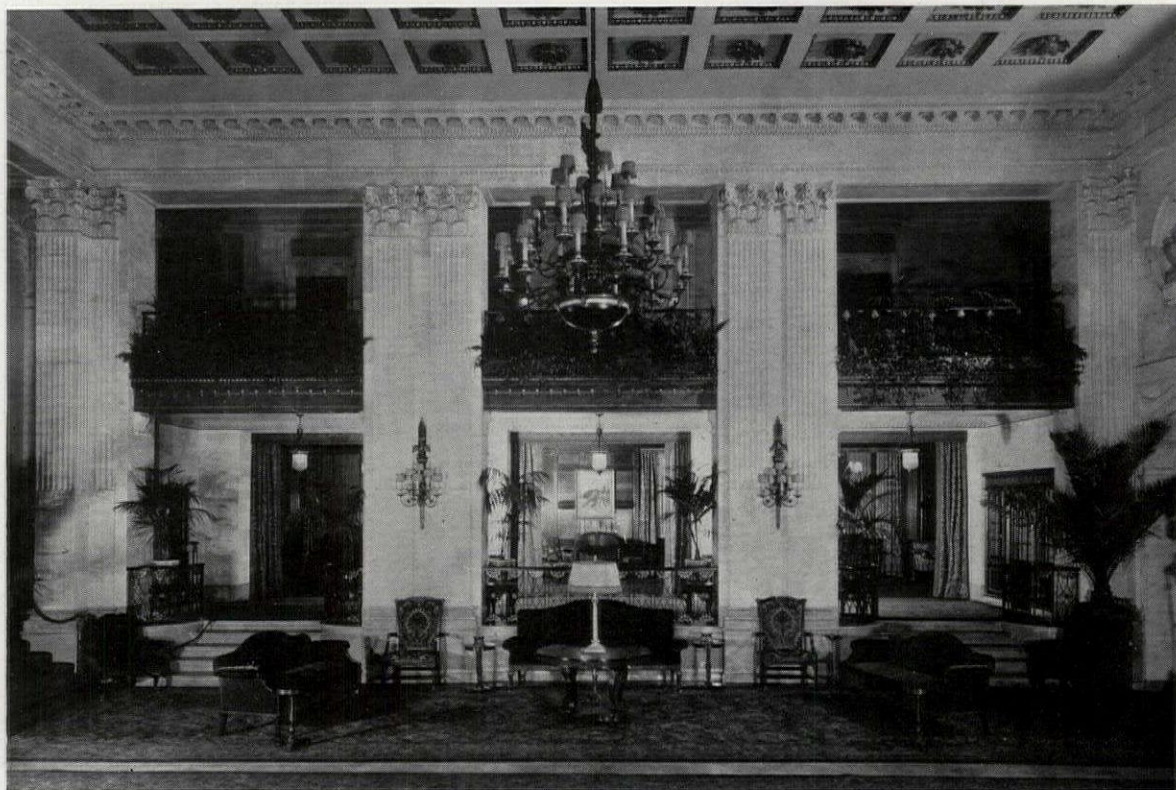
WEST SIDE OF LOBBY
