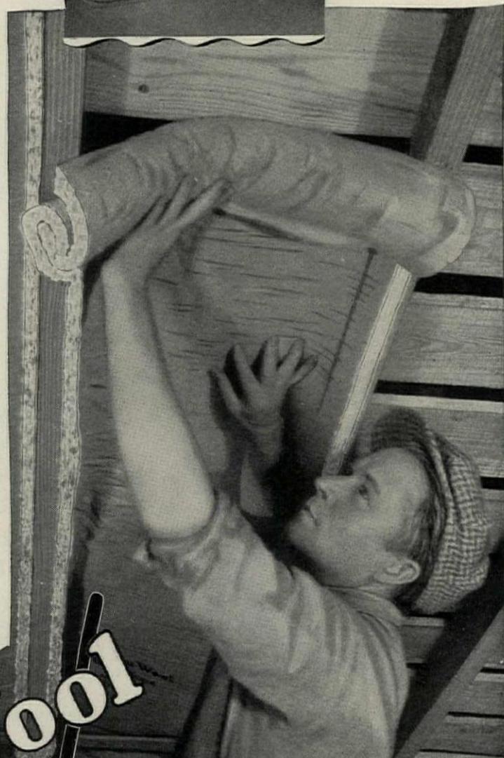
Balsam-Wool can easily be carried through any opening that will admit the body of a workman. Strips of Balsam-Wool cut to proper length in the basement or garage can be carried to the attic by a single workman.
