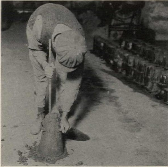
Fig. 11. Rodding the Concrete for Slump Test
