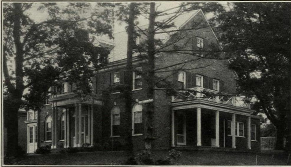
A Cambridge, Massachusetts, home—one of the 5000 homes in New England alone which are heated by Electrol.
