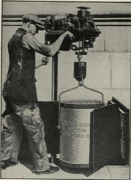
Model E G&G Telescopic Hoist equipment in use at Julia Richman High School, New York. William H. Gompert, Municipal Architect.
