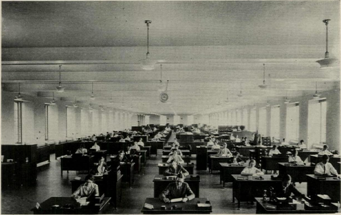
Lighting Fixtures Properly Spaced to Illuminate a Large Open Office Area
