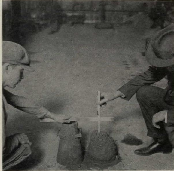
Fig. 12. Measuring the Slump of the Concrete
