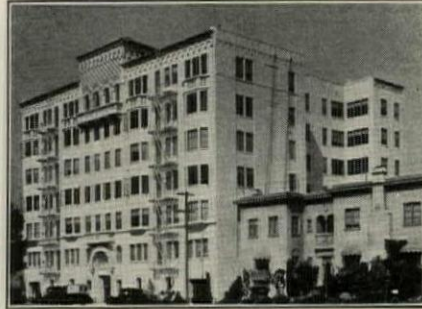
In beautiful Edgemere Manor Apartments, Oakland, Cal., D. D. Stone, architect, STEELTEX puts welded steel fabric on guard in walls and ceilings. STEELTEX for Floors was also used (see right-hand page).
