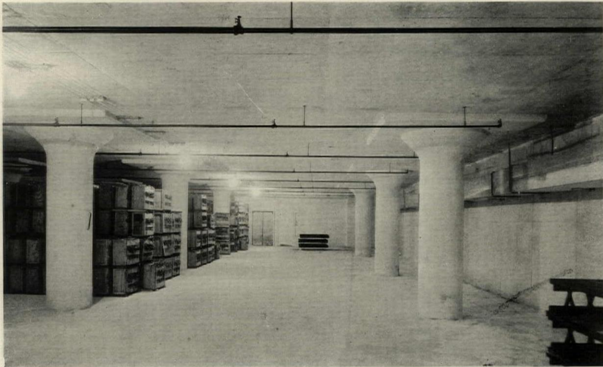
Interior of Great Lakes Terminal Warehouse, Toledo, Showing Construction and Equipment William H. Adams, Architect
