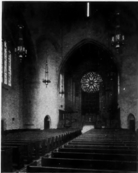
Epworth Euclid M. E. Church, Cleveland Mayers, Murray & Phillip, Walker & Weeks, Associated, Architects
