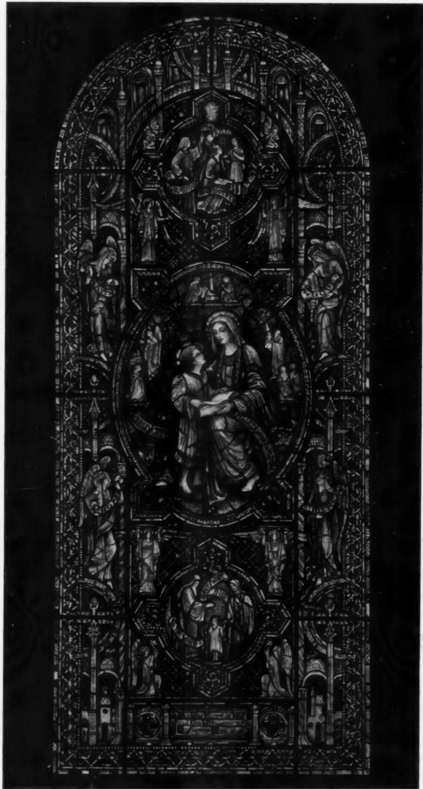
A MODERN STAINED GLASS WINDOW SHOWING THE IRON FRAMEWORK CONFORMING TO THE LINES OF THE DESIGN HENRY LEE WILLET, DESIGNER
