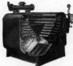
All Spencer Heaters may be hooked up in battery where a flexible supply of heat is needed, or where the total radiation tax is greater than the capacity of a single boiler.
