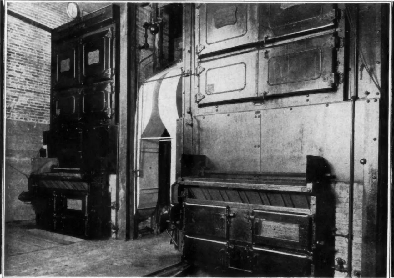
Two "King Coal" automatic mechanical stokers under two 250 hp. Kroeschell Boilers at the Riverside Brookfield High School, Riverside, Illinois.
