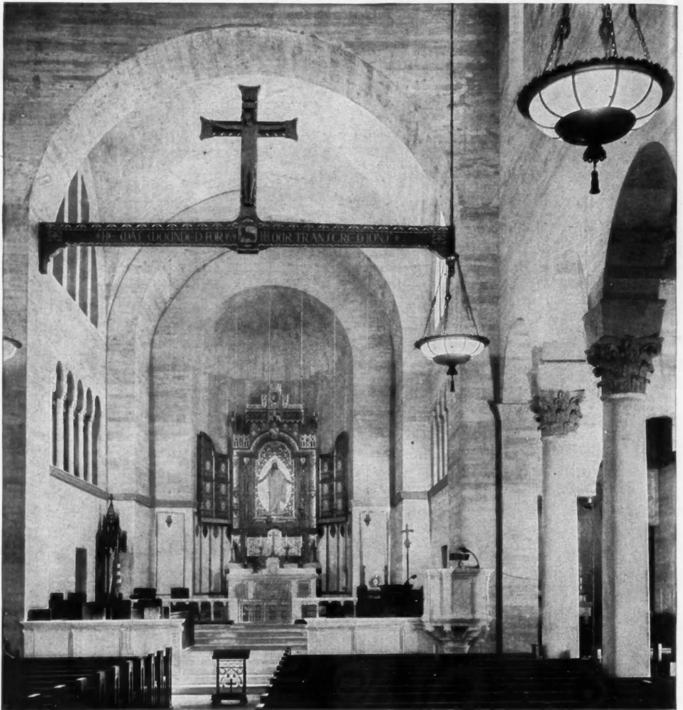
St. John's Episcopal Church, Los Angeles. Both exterior and interior are monolithic exposed concrete—except the facade, which is Tufa. Architectural ornaments were cast in place. Architects: Pierpont and Walter S. Davis, Los Angeles. Con-
