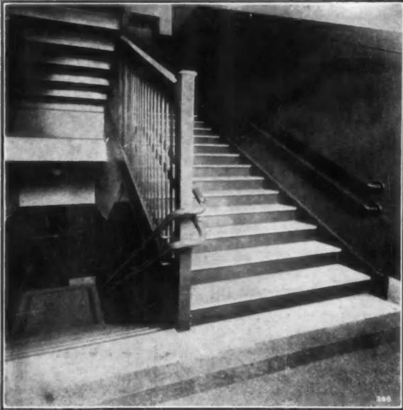
STAIR treads and landings of Alberene Stone have a smooth, but "toothed," surface that neither slips nor grips and gives an equally secure footing wet or dry.
