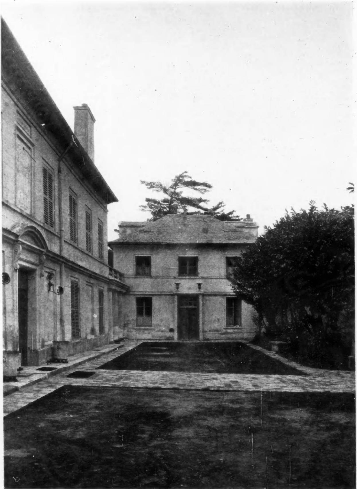
FORECOURT, ST. VIGOR, VIROFLAY, (NEAR VERSAILLES) GUEST HOUSE ACROSS THE COURT
