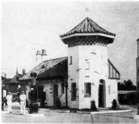
Service and Filling Station, Penn Oil Co., Madison, Wis. Clarence O. Jahn, Designer
