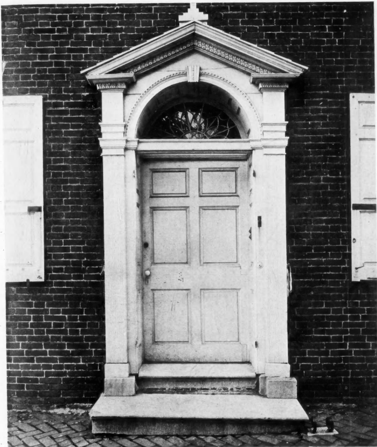
DOORWAY, THOMAS HOUSE, NEW CASTLE, DELAWARE
