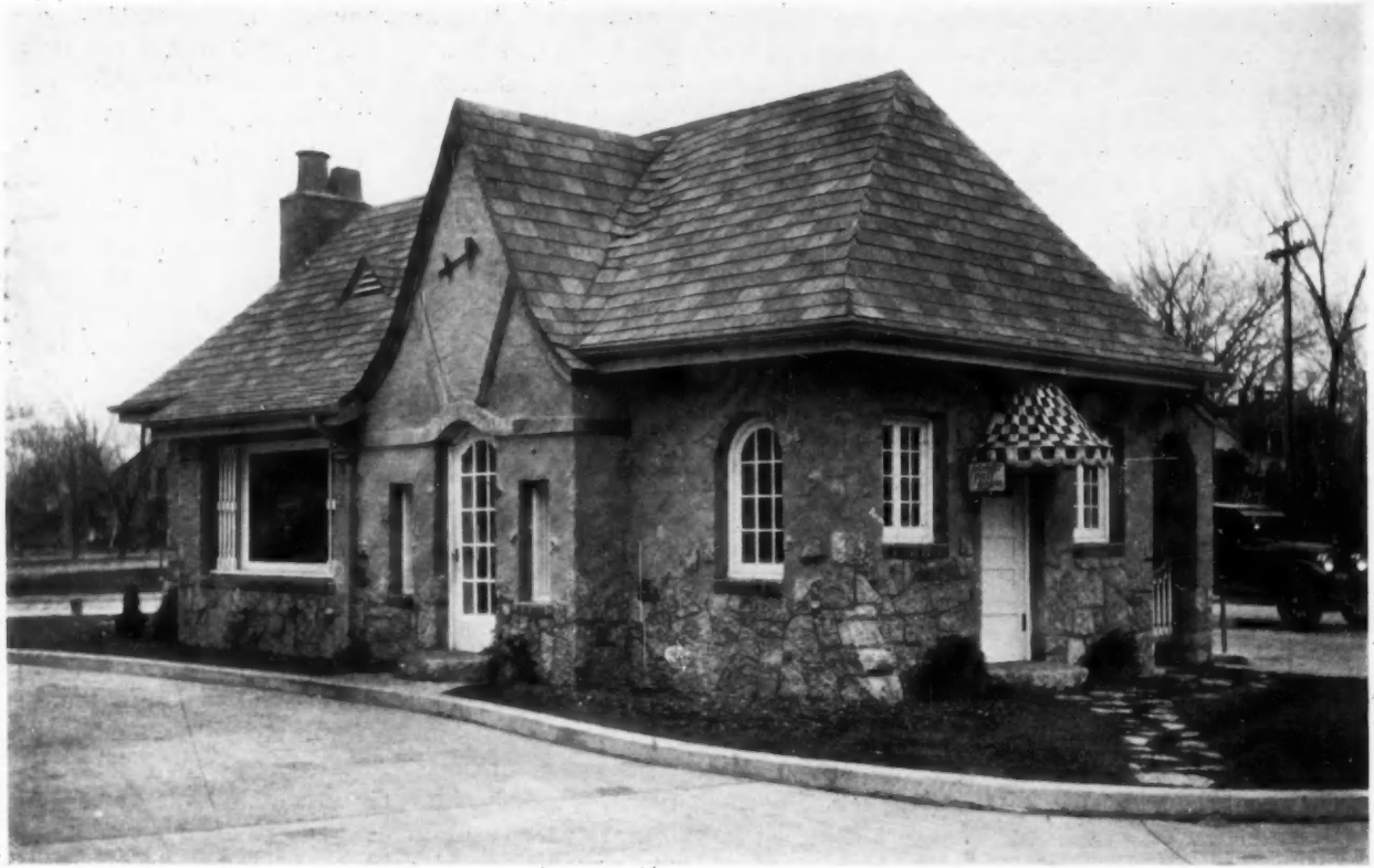
SERVICE AND FILLING STATION, BARKHAUSEN OIL CO., GREEN BAY, WIS. CLARENCE O. JAHN, DESIGNER.
