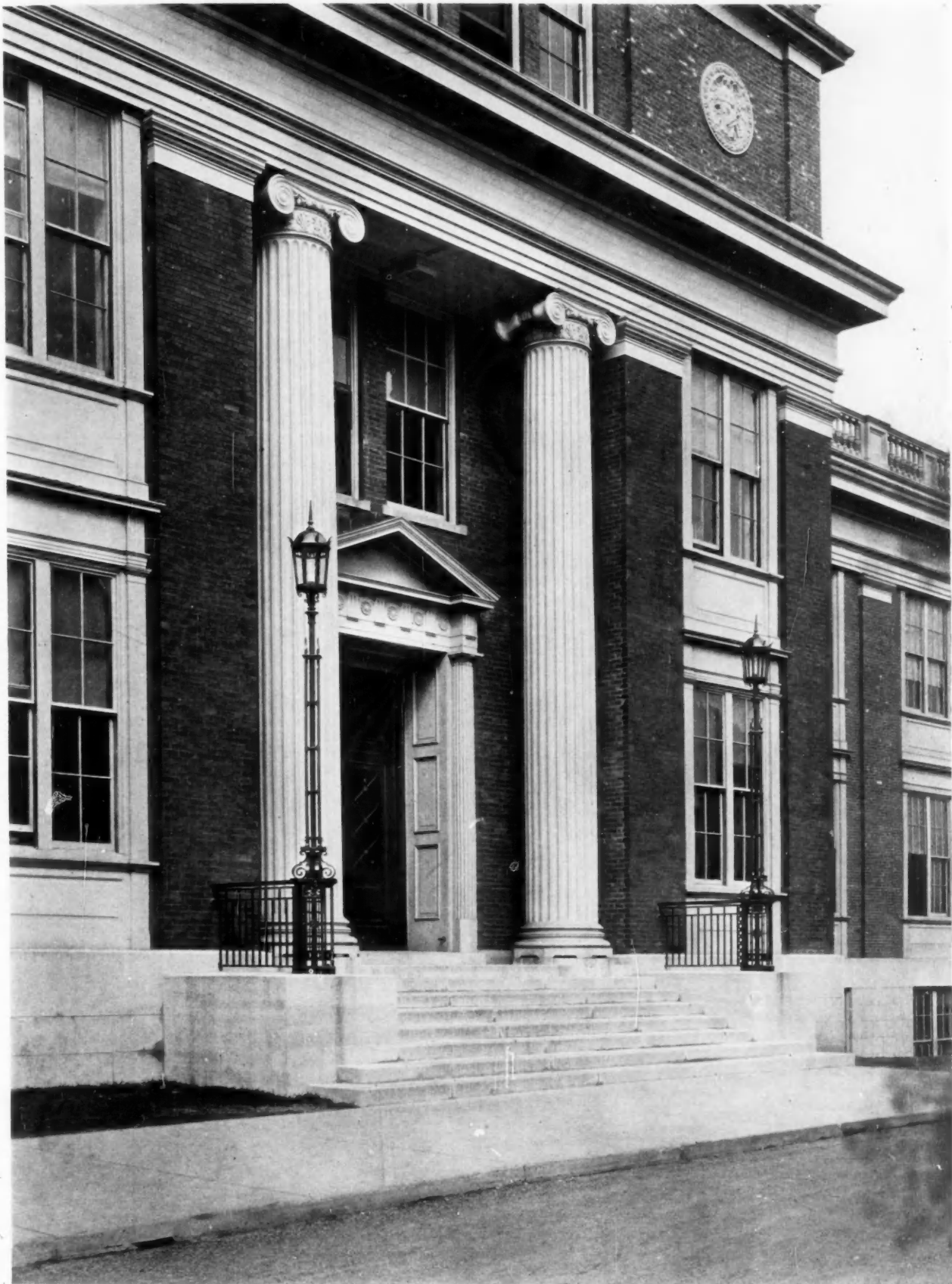
DETAIL, MAIN ENTRANCE, CITY HALL, SOMERVILLE, MASS. RITCHIE, PARSONS & TAYLOR, ARCHITECTS
