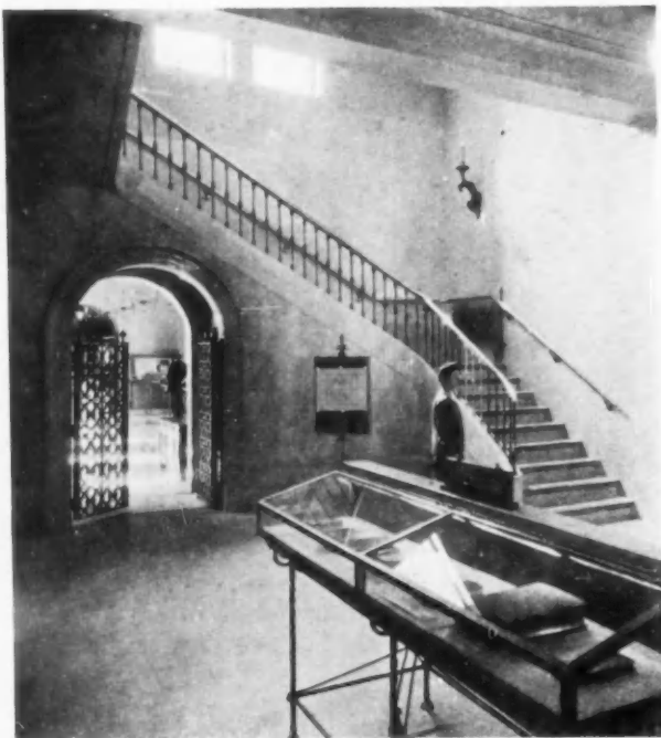
Main Corridor, Third Floor
