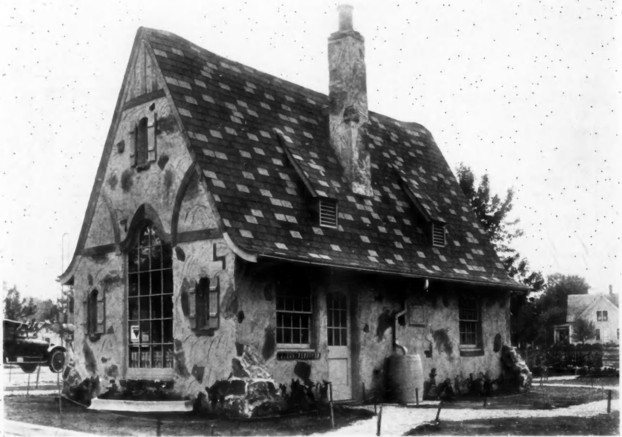
SERVICE AND FILLING STATION, WAUPUN OIL CO., WAUPUN, WIS. CLARENCE O. JAHN, DESIGNER
