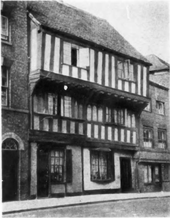
Overhanging Upper Stories Are Often Found in Old Tewkesbury
