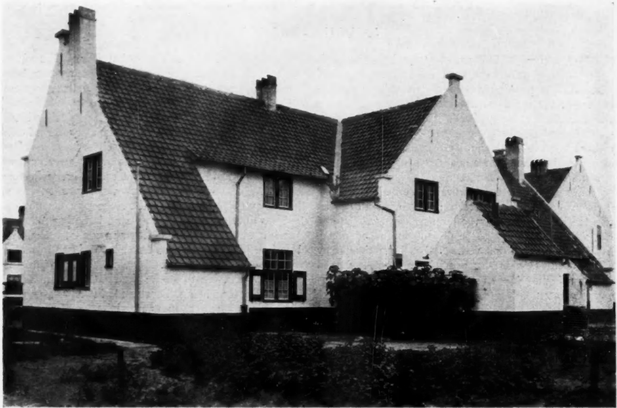
Rear of Cottage, Kalfvaart Garden Suburbs for Working People, Built by the Office des Regions Devastees at Ypres R. Acke, Architect
