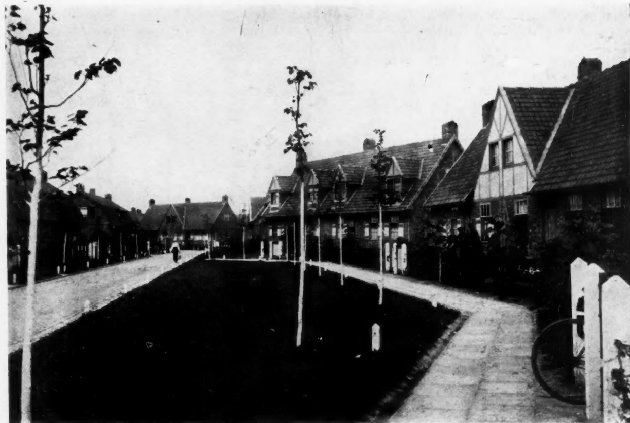
Ligy, Garden Suburb for Working People, Built at Ypres by the O. R. D. H. De Bruyne and Ralph Verwilghen, Town Planners
