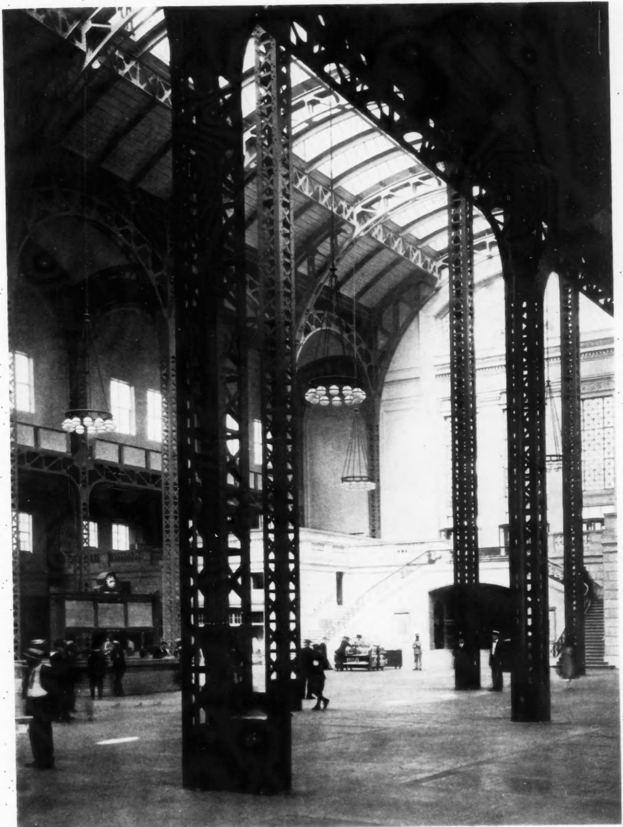
SECONDARY CONCOURSE CHICAGO UNION STATION GRAHAM, ANDERSON, PROBST & WHITE, ARCHITECTS
