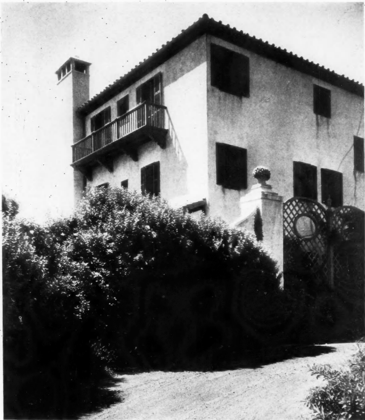
Driveway to Entrance, The Villa Maria, Southampton, N. Y.
