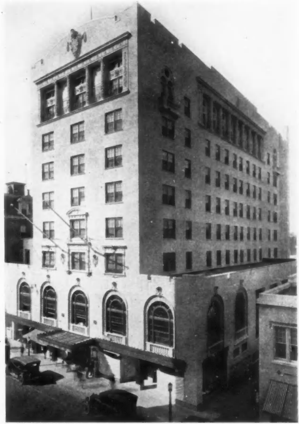
San Juan Hotel, Orlando, Fla. William L. Stoddart, Architect
