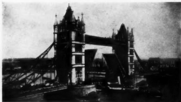
Fig. 7. Tower Bridge, London
