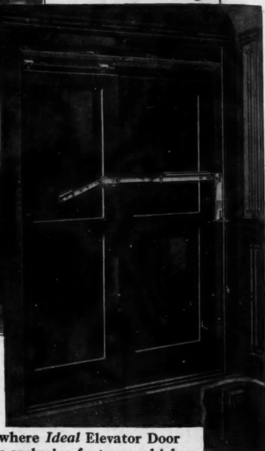
Electric Door Controller with cut-out switch in pit at bottom of elevator shaft. Pulley and weight—for controlling switch wires—are located in pent house.
