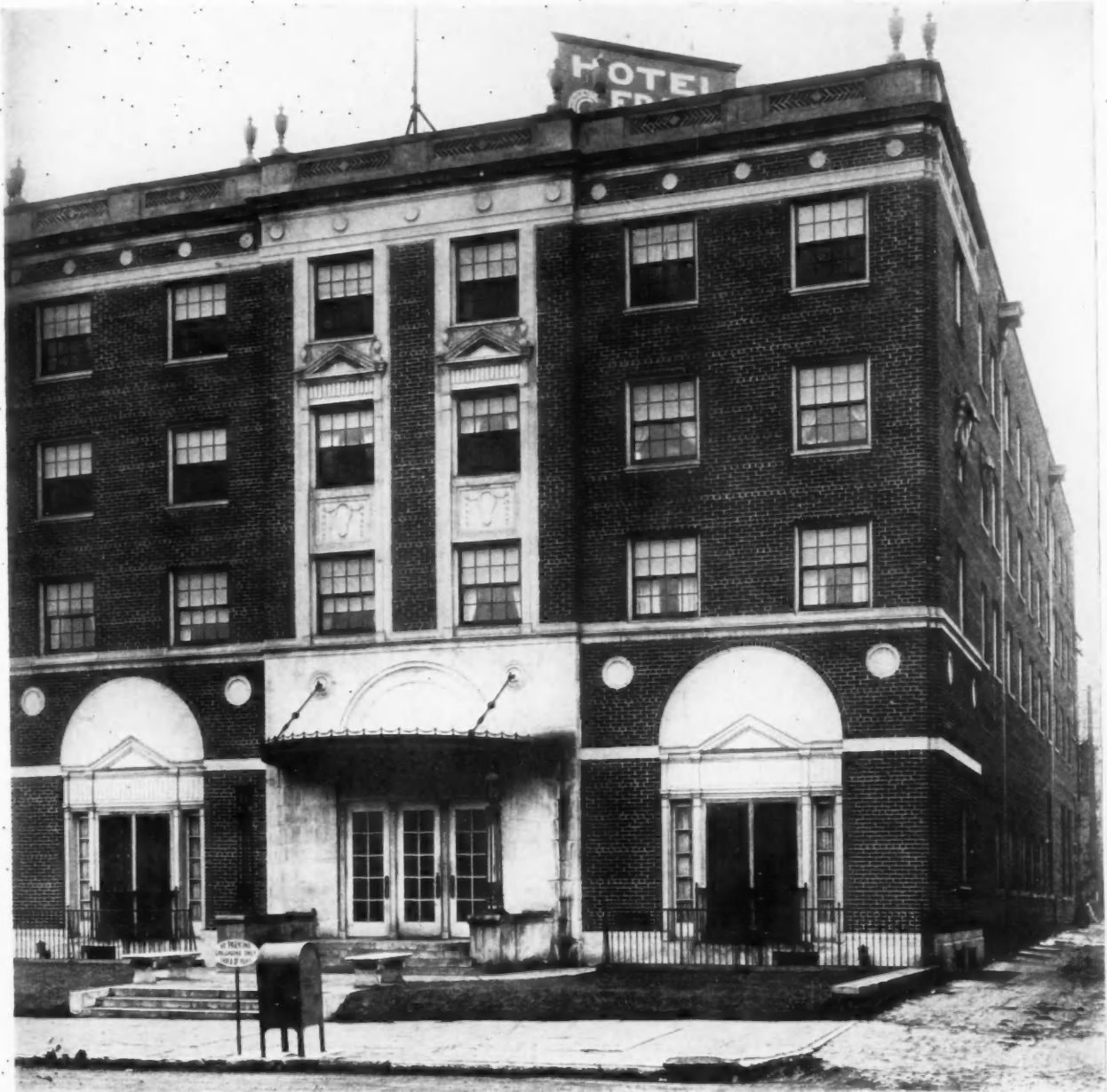
HOTEL FRANCE, PARIS, ILL. JOHNSON, MILLER, MILLER & YEAGER, ARCHITECTS
