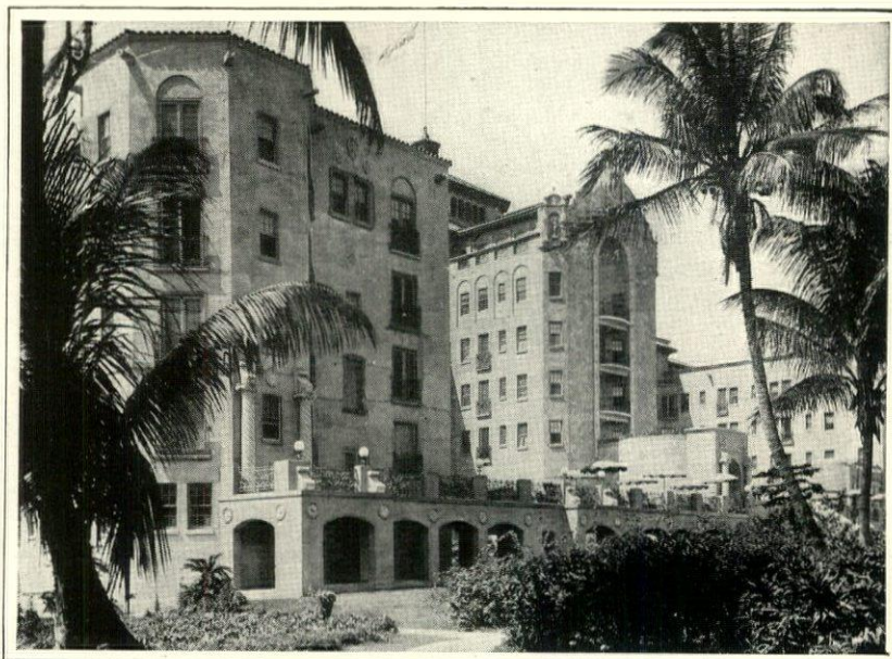
NEW COLONIAL HOTEL, Nassau, Bahamas: Kenneth Murchison, New York City, Architect; C. F. Driggs, Inc., New York City, Jobbers; Gustave Staats, New York City, Plumber
