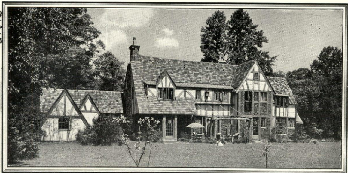
Home of WALTER PLEUTHNER, Architect, Scarsdale, N. Y.
