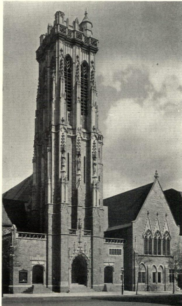
"Christmas Tower," Emmanuel Church, Baltimore Woldemar H. Ritter, Architect
