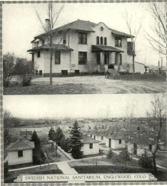
SWEDISH NATIONAL SANIARIUM, ENGLEWOOD, COLO. Mountjoy & Frewen, Denver, Colo., Architects J. W. Hancock Electric Co., Denver, Colo. Electrical Contractors
