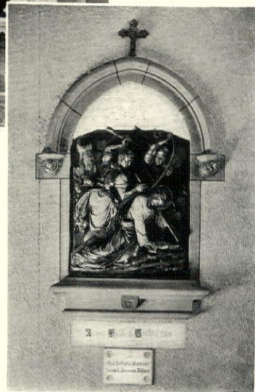
View of wall and station showing fine texture obtained by the use of Morene.
