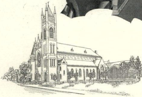
St. Mary's Church at McSherrystown, Pa. 3,800 square feet of Armstrong's 6-mm. Brown Battleship Linoleum, No. 20, installed in the Auditorium. Cemented over deadening felt.
