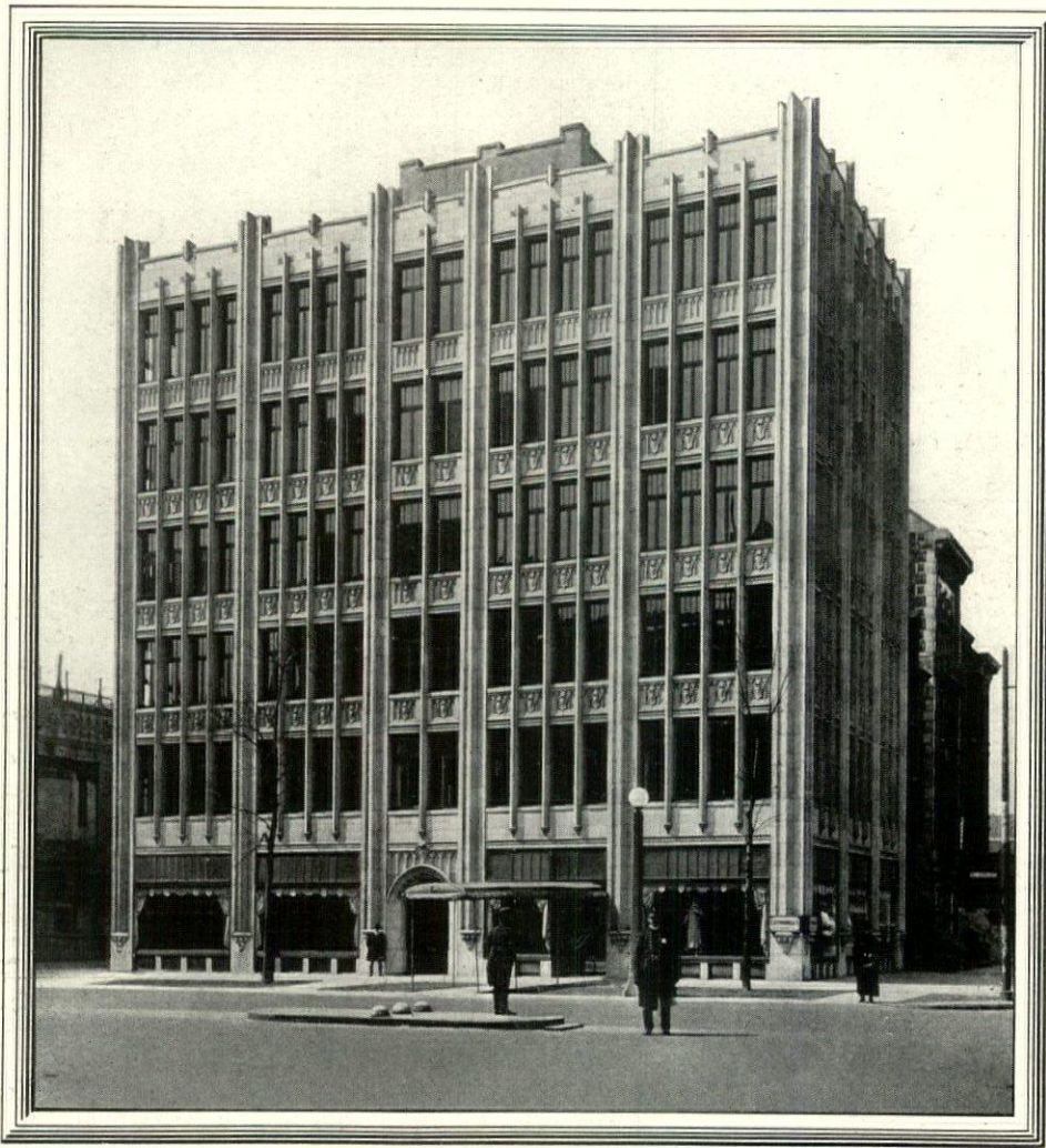
Building at Michigan and Chicago Avenues, Chicago — Entire Facing of Cast Stone Robert T. Newberry, Chicago, Ill., Architect. Ridenour & Erickson, Chicago, Contractor
