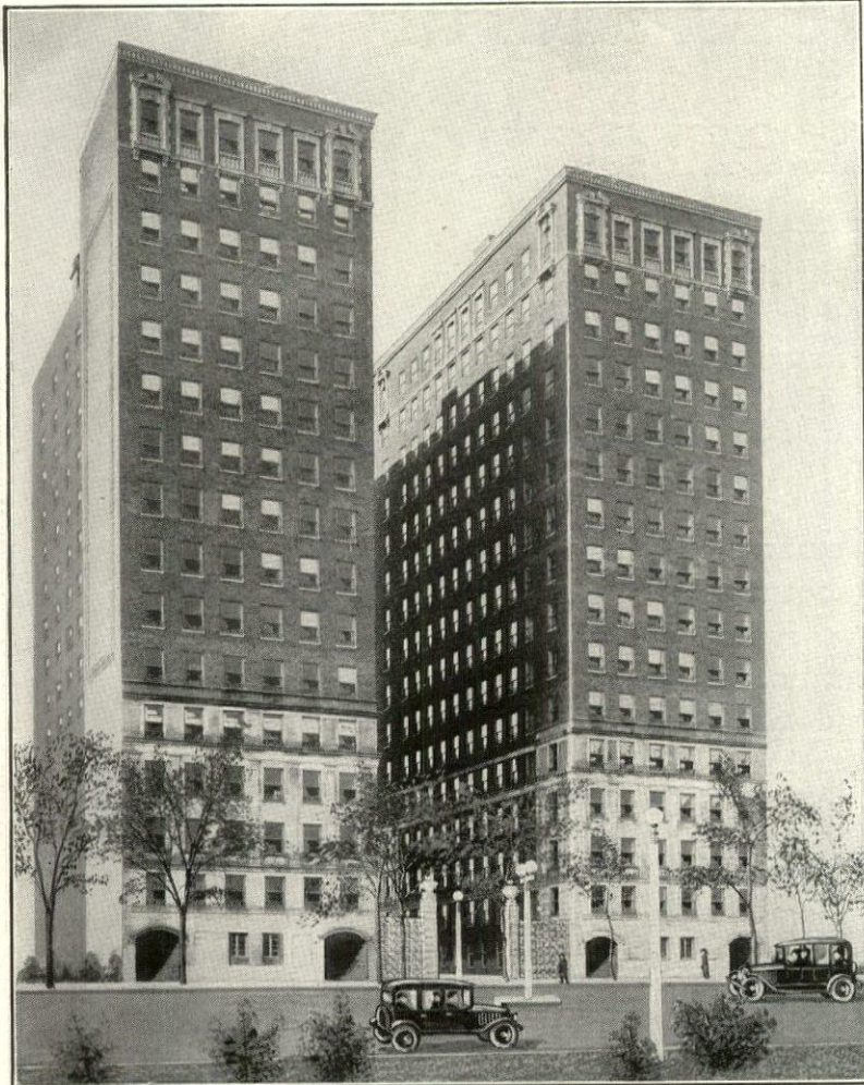
The Sheridan Lake, Chicago—co-operatively owned apartments of six rooms with three baths each. Heated by four No. 20 Simplex Smokeless Steel Boilers of 10,000 sq. ft. capacity each. Walter W. Abschlager, Chicago, architect. Hanley & Co., Chicago, heating contractor.
