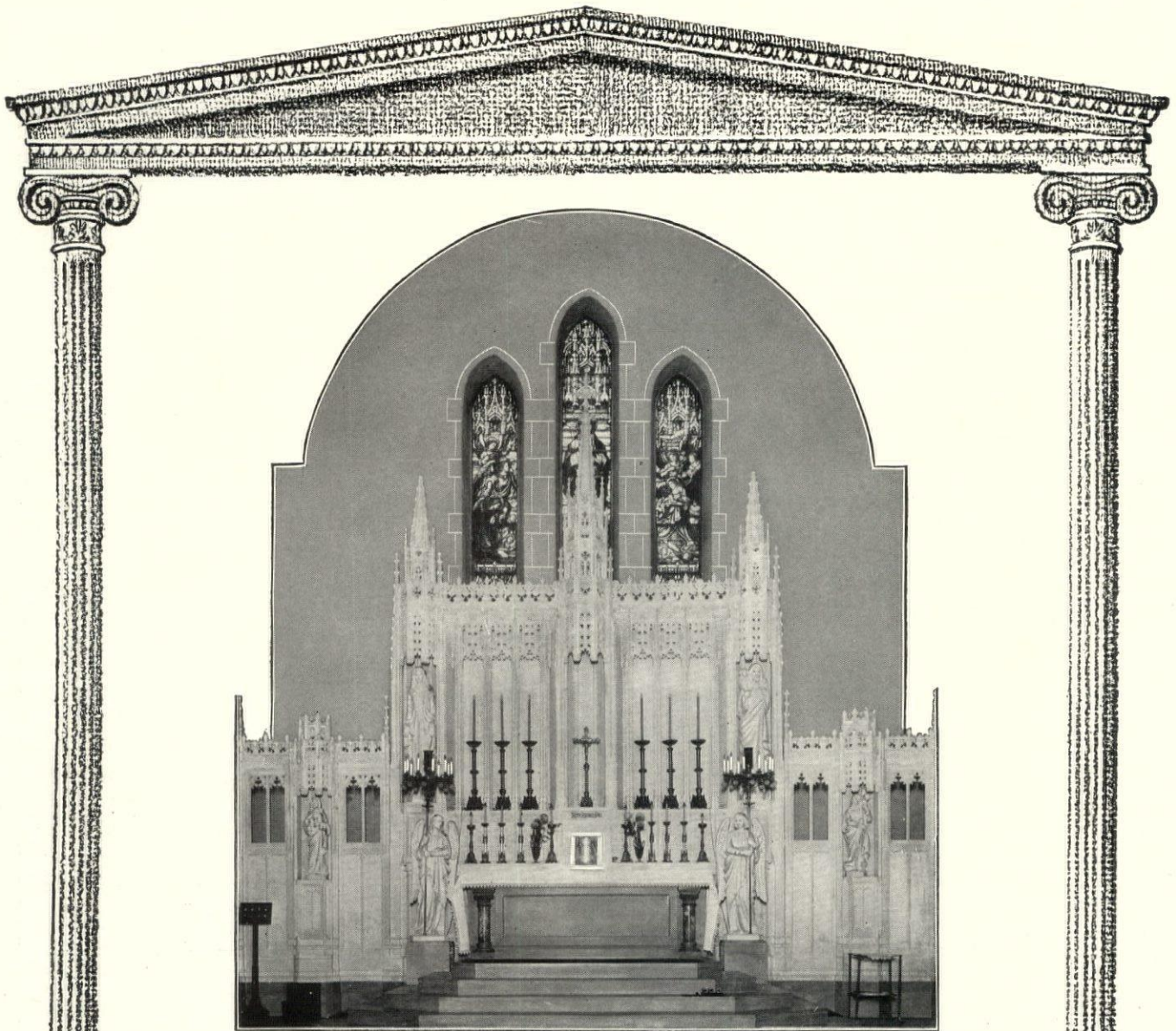
American Cream White Lens Altar with Pink Tennessee Marble Steps and base, in Holy Name Church, Philadelphia, Pa. Maginnis and Walsh, Architects. J. Hegerty, Marble Contractor
