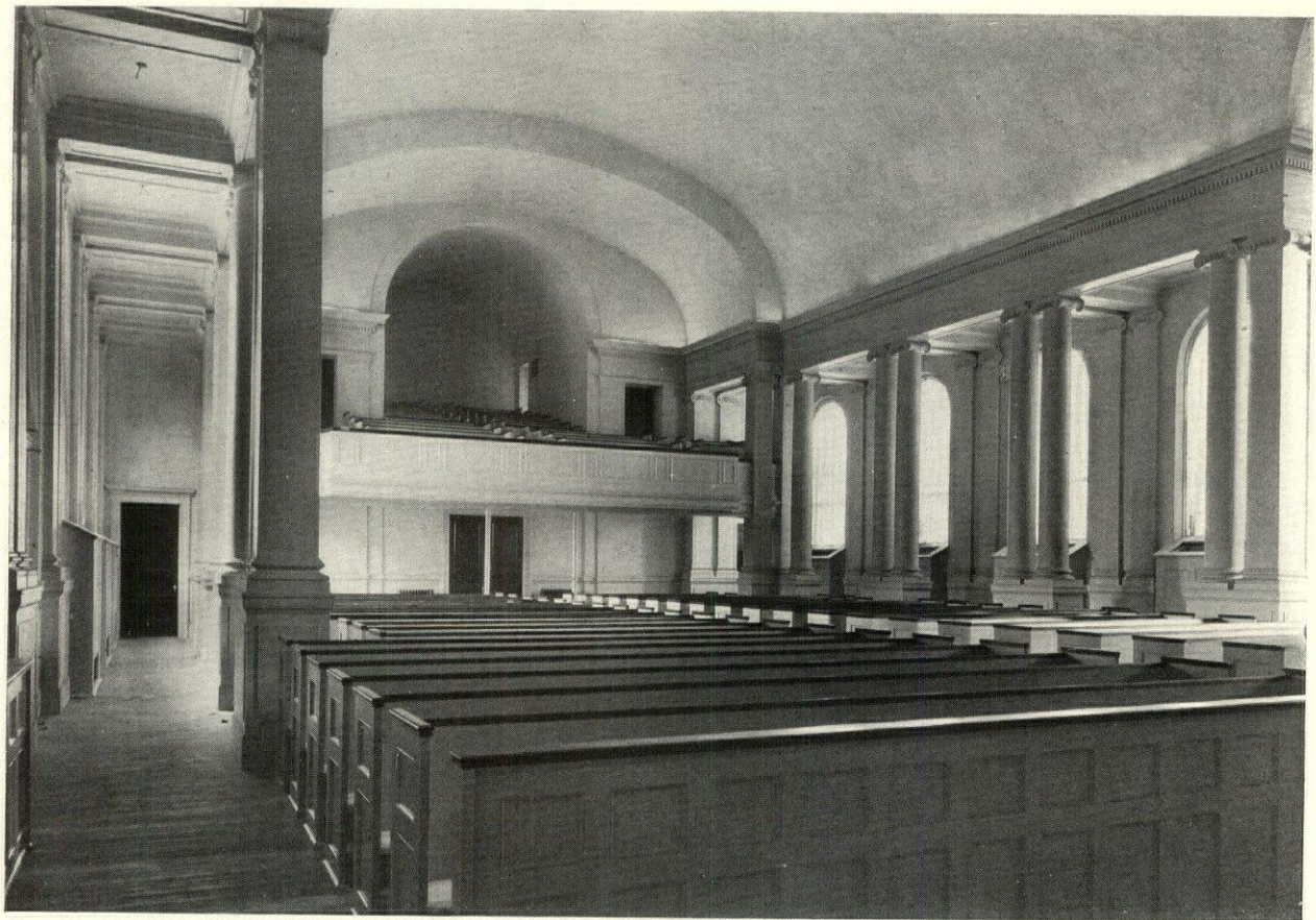
Auditorium, Looking Toward Narthex, Congregational Church, Wellesley, Mass.
