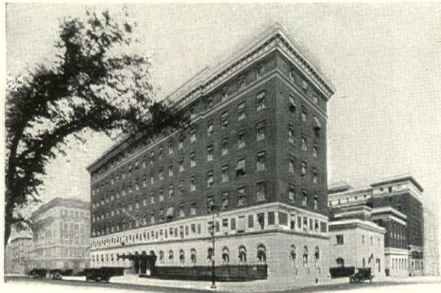
Mt. Sinai Hospital, New York City, equipped with two Pfaudler Glass Lined Laundry Chutes. Architect, Arnold W. Brunner, New York City.
