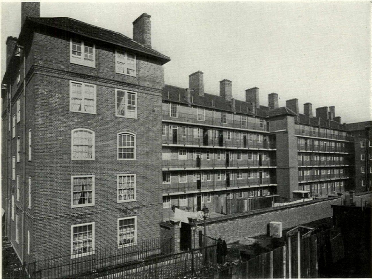
Court View of Geoffrey House, Tabard Garden Estate, London G. Topham Forrest, Architect to the London County Council
