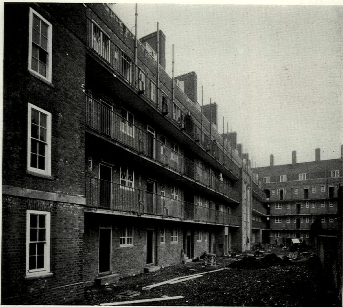
Rear View of Bullen House Showing Balconies Giving Access to Tenements G. Topham Forrest, Architect to the London County Council
