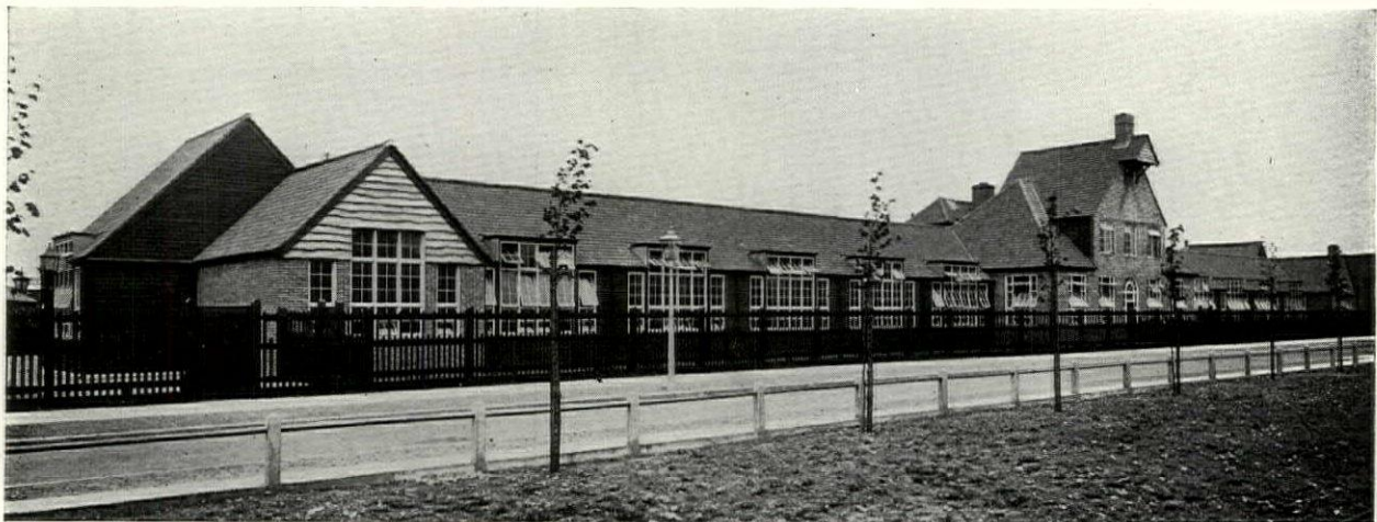
Elementary School, Bellingham Estate of the London County Council G. Topham Forrest, Architect to the Council
