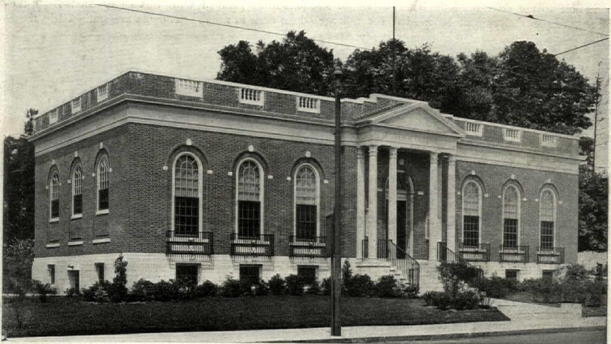
Branch Library for City of Boston, West Roxbury, Mass. Oscar A. Thayer, Architect
