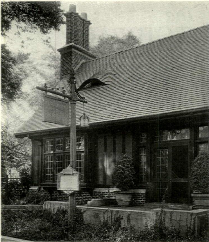
Detail of Front, Easthampton Free Library
