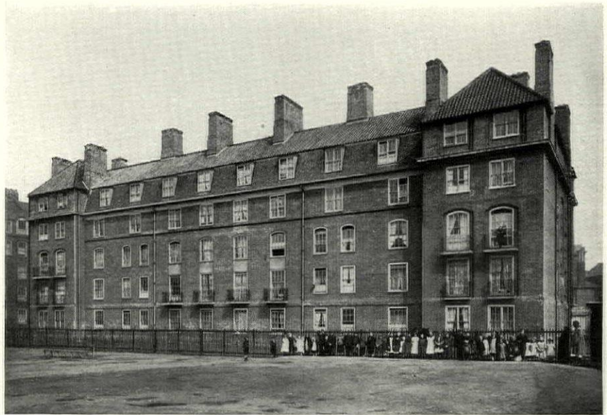
Harbledon House, from Recreation Ground
