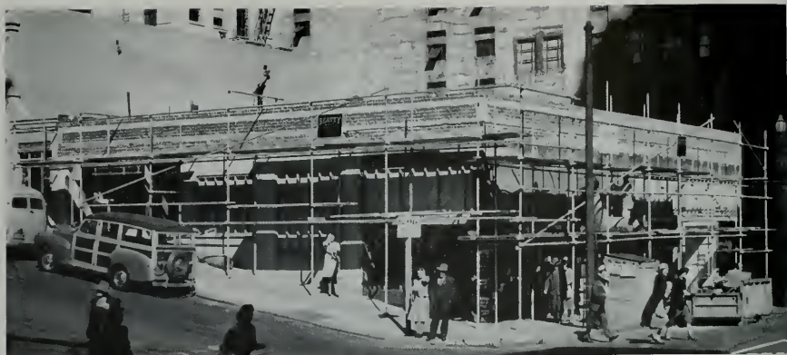
Aluminum scaffold provides level working platforms and minimum sidewalk obstruction for this sloping San Francisco work site Moulin Studio Photos
