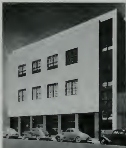
Watsonville: Ariston steel sash with stainless steel trim on ground floor and stair well, and stainless steel doors and entrance.
