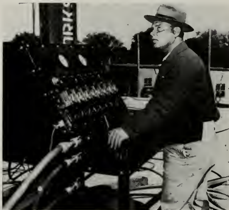
Ken Hewitt, SRI engineer at control for lifting concrete slabs. ▶
