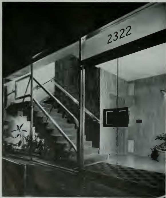
Main portal detail showing veneer application of Roman brick laid vertically with stacked joints to give illusion of greater expanse. Stairway and floor are terrazzo finished. Area is enclosed in 9 ft. high plate glass panels inset with double glass doors.
