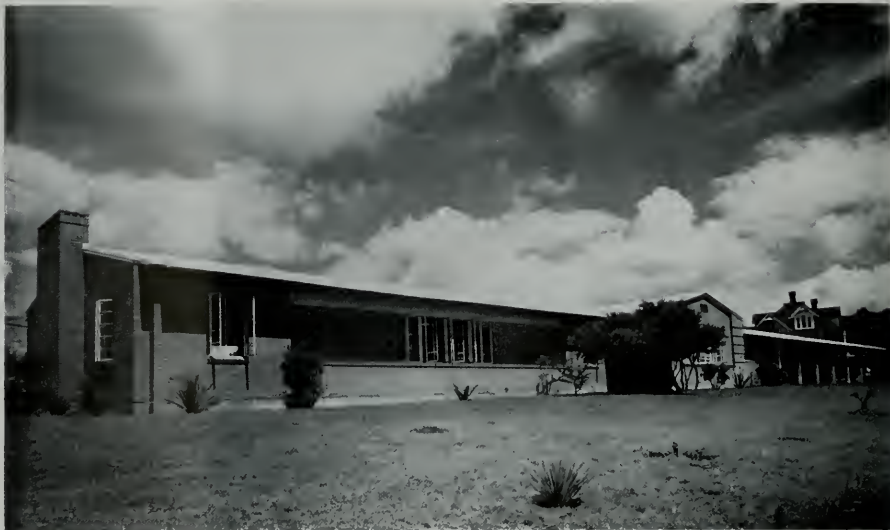
One of fourteen Laboratory Buildings which comprise the Southwest Research Institute at San Antonio, Texas.
