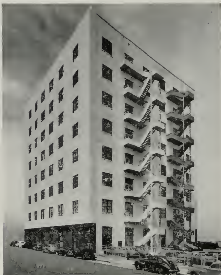
San Francisco: Ariston stainless steel trim and windows on stair well, stainless steel entrance and door, steel stairs and fire escapes.
