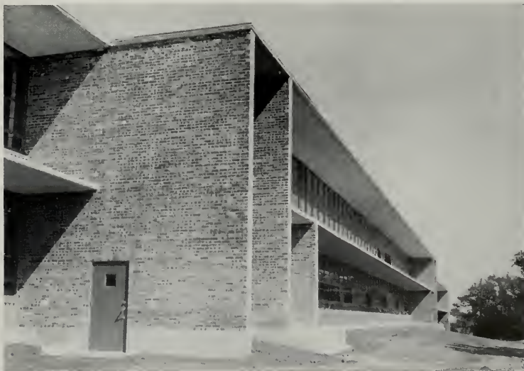
Partial view of finished Trinity University Administration Building.
