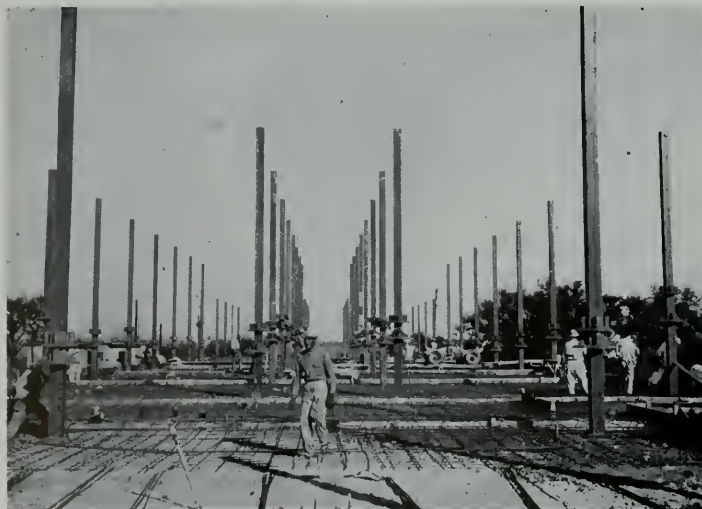
◀ Hydraulic Lifting Unit atop steel column.
