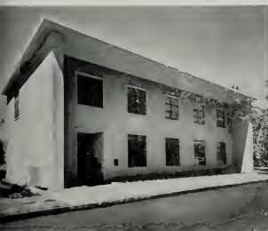
Sanford: Ariston steel sash, steel stairs and fire escape, stainless steel entrance and doors.
