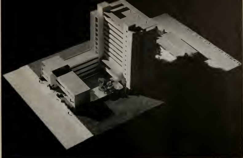
OVERHEAD VIEW of entire project. Number of stories can be increased without blocking light from the utility side of the ward building.
