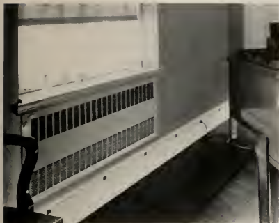
ELECTRICAL OUTLETS every 18 inches around the walls provide maximum opportunity to plug-in desk lamps, dictating machines, fans, check protectors and other electrical office equipment.
