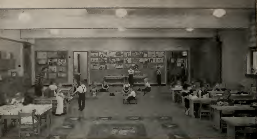
THE Floor of the Kindergarten is asphalt tile over concrete slab. Side wall is pumice block construction covered with acoustic material.
