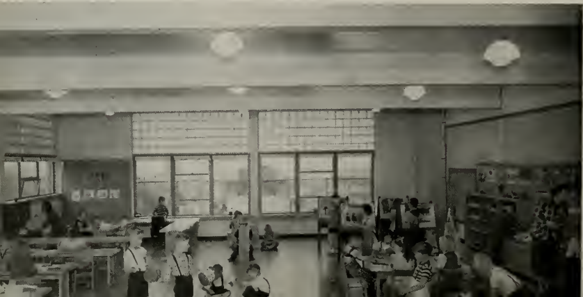
THE Kindergarten has laminated glued up wood girders to support the roof. These are not cased, only painted.
