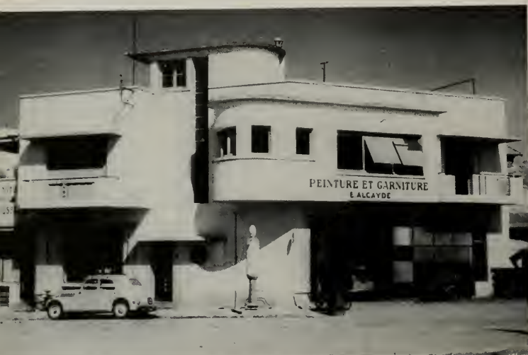
AUTOMOBILE painting and accessories shop in Rabat, built of concrete and masonry at a cost of $7200 in 1936 BORIS NEPO, Architect.
