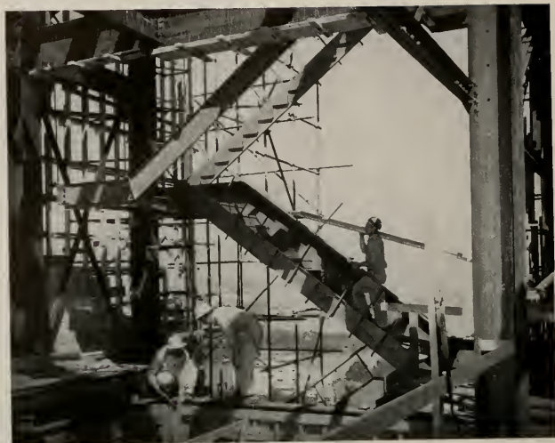
Installation of form work preparatory to pouring concrete on 14th floor.
