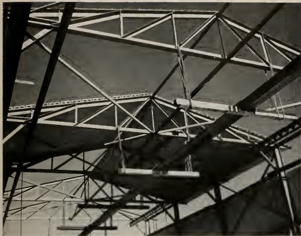
Roof trusses with Strestcrete roof slabs in place to be grouted.
