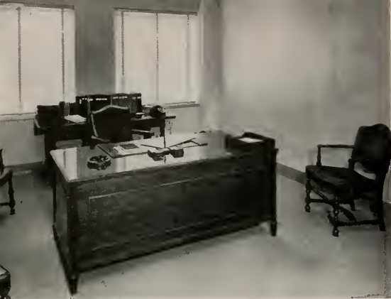
View of typical outside of- fice; wall on the right is a movable partition which may be removed to enlarge office by a simple disassem- bly operation involving no destruction. All components of the wall are reusable.
