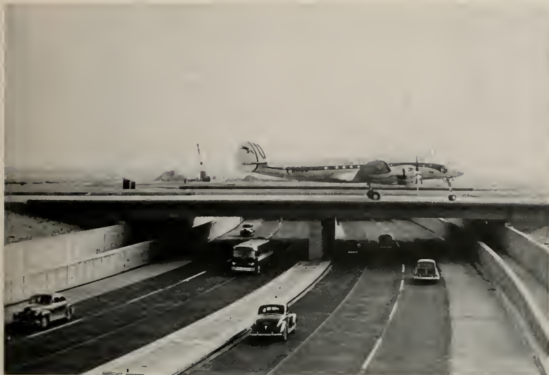
AN Air France Constellation taxis over the world's first roadway underpass built to permit the simultaneous movement of aircraft and surface vehicles at New York's International Airport. The Port of New York Authority Photo.
