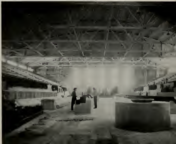
INTERIOR before maple floor is laid. Shows amphitheatre plan with permanent bleacher seats high above floor level.
