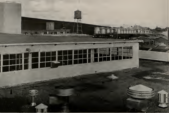
Pent House contains a lunch and recreation room which overlooks the hillside tank farm which supplies the factory's point and varnish departments.
