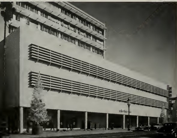
First Three Floors of the eastern wing are occupied by a well known New York Department Store.
