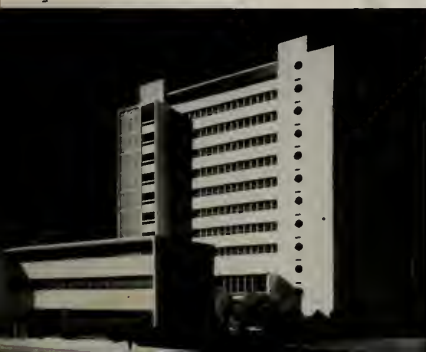
UTILITY FRONT (North Side). Courtyard onto the street giving easy access to all parts treatment wing and utilities.
