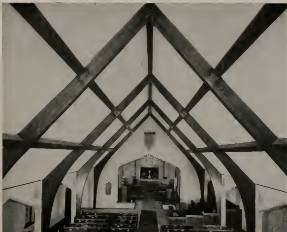
Seattle's St. James Lutheran Church by Architect C. F. Nelsen offers still another evidence of individual designing of church interiors with glue laminated arches. Arches form both roof and wall support.
