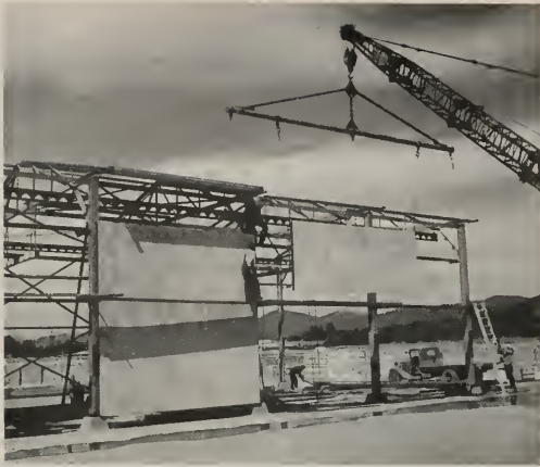
Panel of tongue and groove siding being lifted into place by crane. Section span is 16 ft. 3 in. and is 6 ft. 8 in. high.
