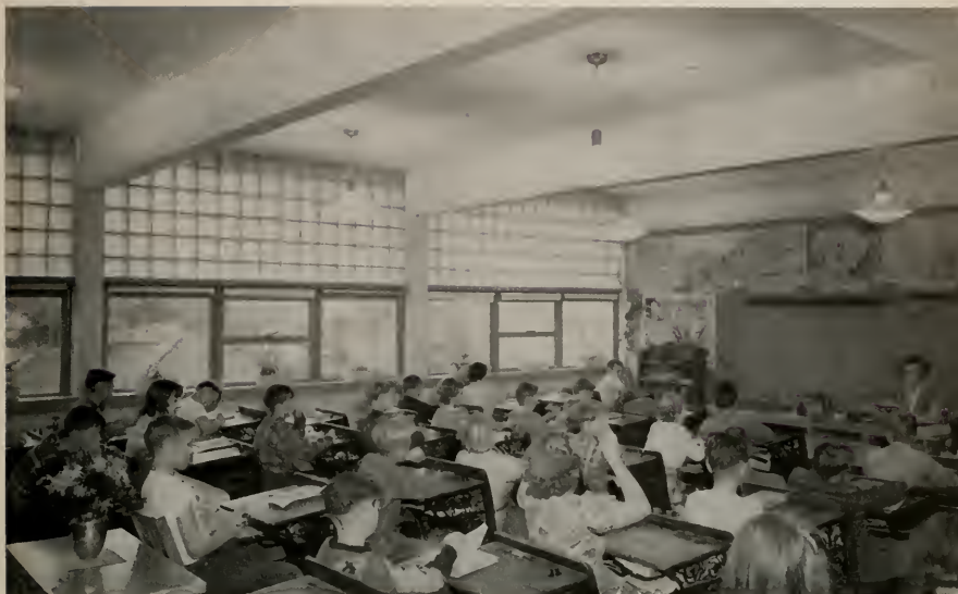
A typical classroom showing the simplicity of the roof construction using laminated glued up girders and exposed concrete block walls.
