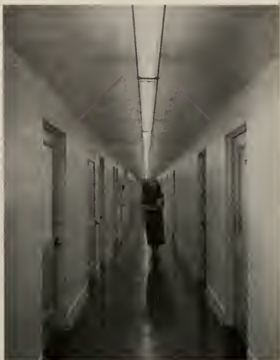
ABOVE VIEW shows corridor lighting with ceiling mounted louvered unit. Glass side panels give even distribution of light on ceiling and side walls.
