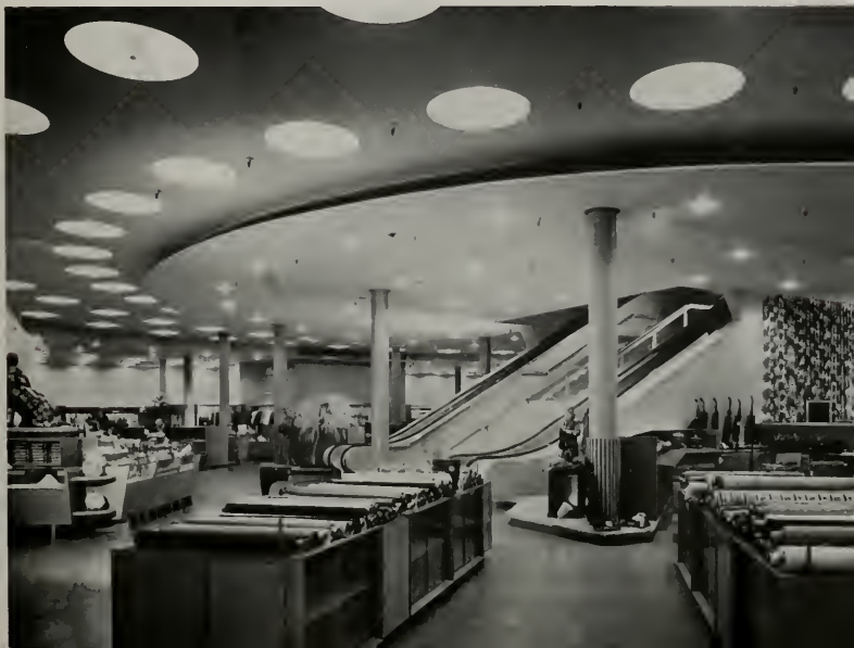
ROOF and MAIN FLOOR are connected with two escalators and 40' stairway.
