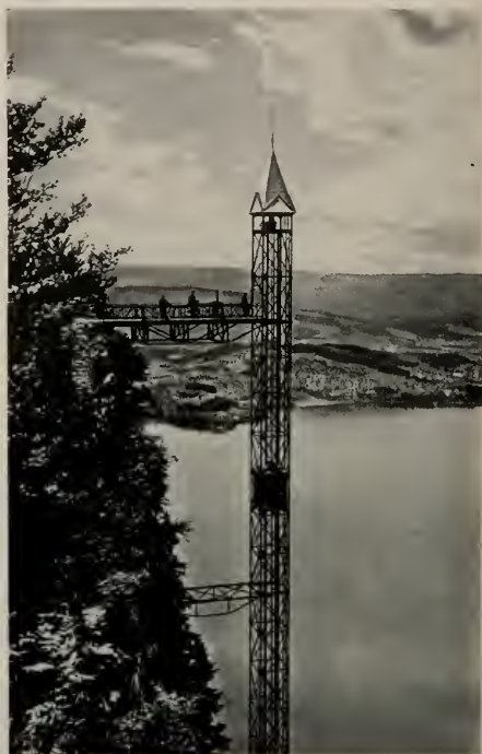
Unique indeed is the open air passenger elevator at Burgenstock which carries people from the high mountain cliffs to the lake shoreline below.
