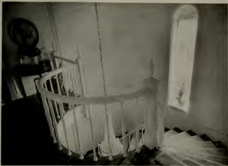
STAIRWAY, "PICKFAIR" RESIDENCE, BEVERLY HILLS, CALIFORNIA
