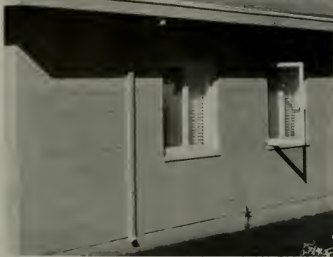
DETAIL OF HAMILTON FIELD HOUSING UNIT, SHOWING BASALITE LIGHTWEIGHT CONCRETE UNIT CONSTRUCTION
