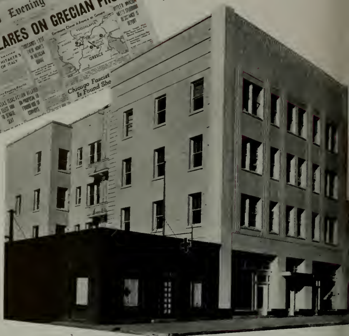
Before and after views of the Gazette Building, Reno, Nevada. Finished in N. Clark & Sons' Adhesion Type Ceramic Veneer. DeLongchamps & O'Brien, Architects. Walker Boudwin Construction Co., Contractors. William Ward Co., Ceramic Veneer Setters.
