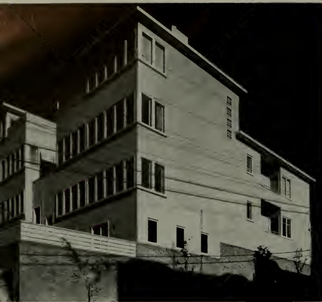
VIEW OF MOROSIN-ARRIGONI FLATS LOOKING TOWARDS THE BAY. NOTE ABUNDANCE OF WINDOW SPACE.
