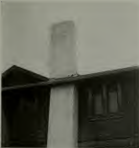
Chimney broken and twisted at roofline on J. W. Bailard Estate, 12 miles south of Santa Barbara on U. S. Highway No. 101.
