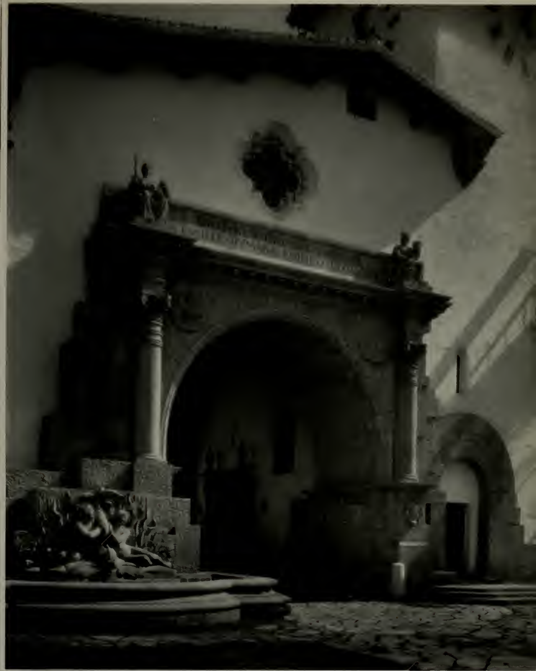
MAIN ARCH OF THE SANTA BARBARA COUNTY COURT HOUSE, SANTA BARBARA, CALIFORNIA William Mosser Company, Architects
