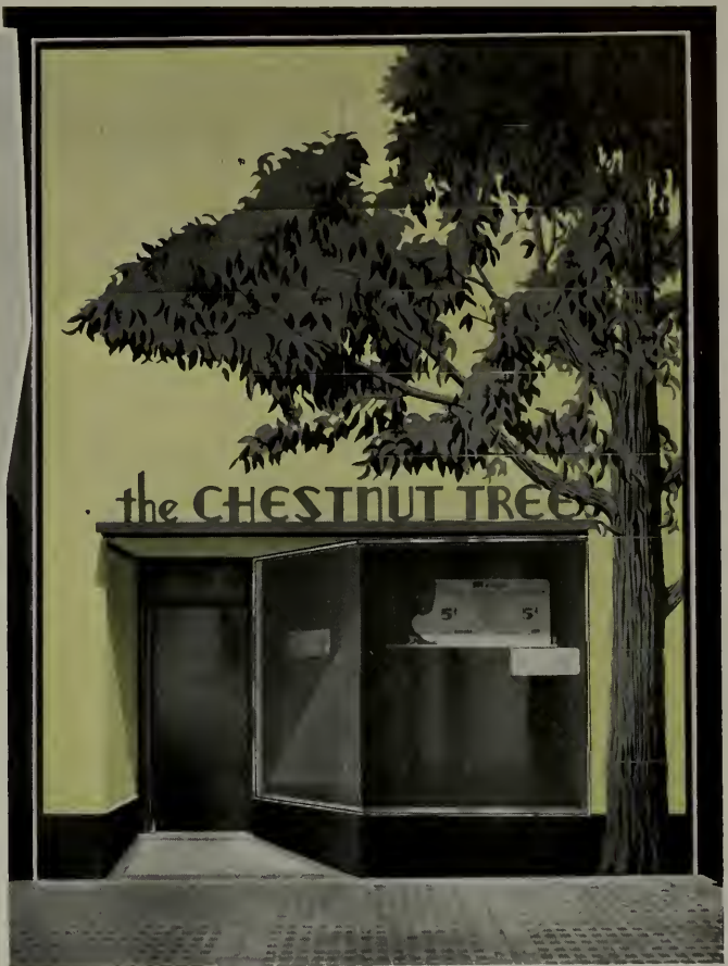
FRONT DESIGNED BY Frank Stauffacher; general contractors, William C. Tait, Inc.; both of San Francisco; enameling by the Ferro Enameling Company, Oakland, California on U·S·S VITRENAMEL Sheets; furnished and installed by Frank Allen Ferro-Porcelain Constructors, San Francisco and Los Angeles.
