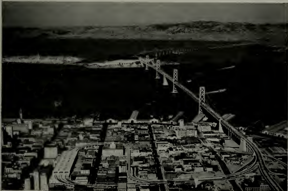
San Francisco Bay Bridge, showing route of interurban trains from Terminal Station (left foreground). At end of the four towers traffic is through a 1000-foot tunnel on Yerba Buena Island, then over a cantilever bridge to the East Bay cities. Treasure Island is seen at the left of Yerba Buena.
