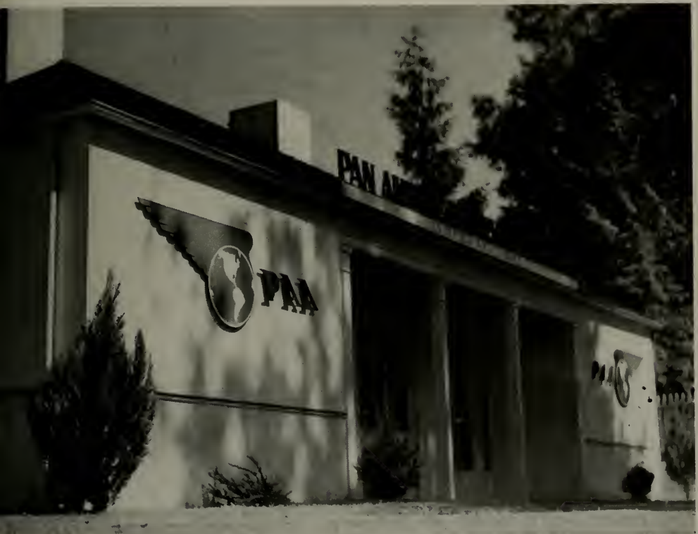
PAN-ALASKA AIRWAYS TEMPORARY BASE, SEATTLE, WASHINGTON Seattle sea plane passenger service base is located on Lake Washington. Built of waterproof plywood painted a light sandstone color, the building is intended to fill the needs of the Airways only temporarily. When regular passenger planes supplant the present sea planes the base will be moved to another location. Interior walls, with one exception, are temporary and may be moved as desired. Thus, with a few alterations, the building may become an attractive residence.
