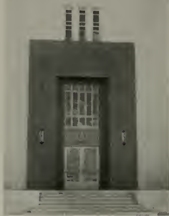
This striking entrance to the Pondera County Court House, Conrad, Montana, is
