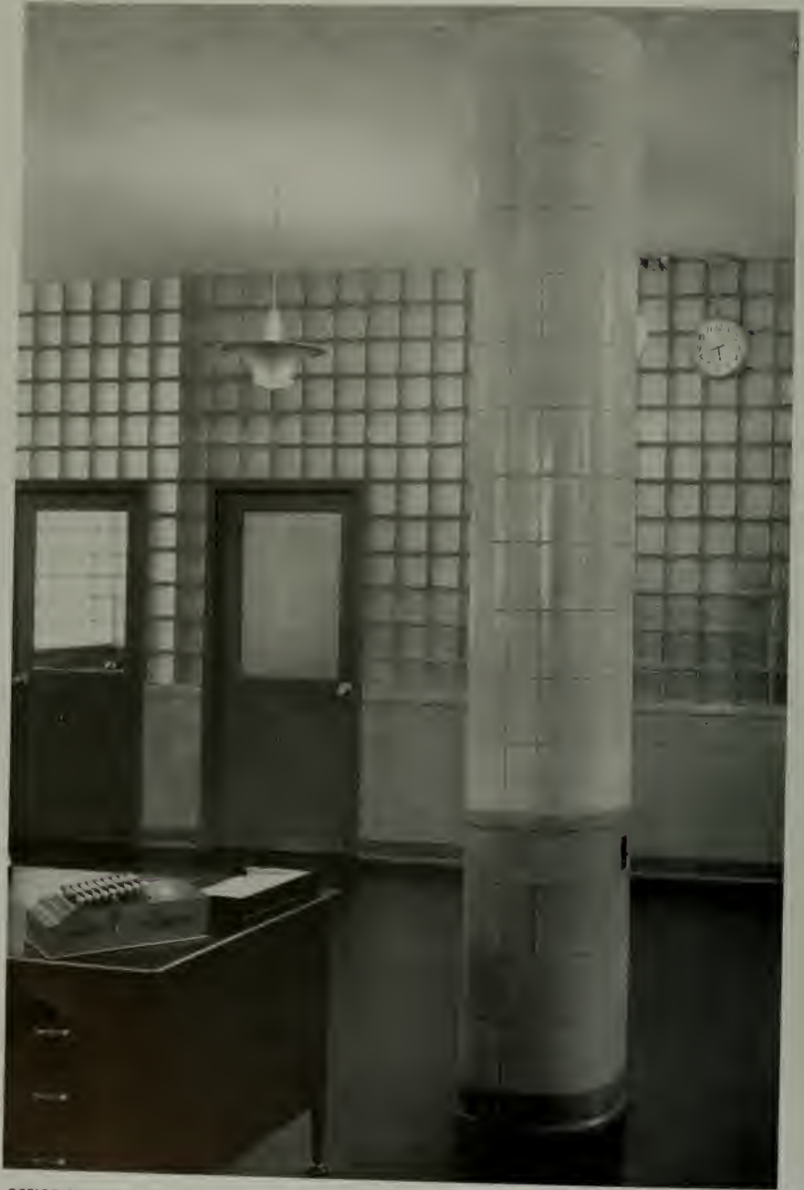
OFFICE BUILDING OF OAKLAND MANUFACTORY—AN INSIDE CORRIDOR WITH WAINSCOT OF KRAFTILE WALL UNITS IN LIGHT GREEN, WITH BASE OF DARKER GREEN. ABOVE THE WAINSCOT THE COLUMN IS SHEATHED IN NEW IVORY.
