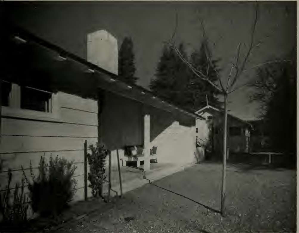
These two houses, one for the grown son and his guests, were designed for vacation use but are adequate for all year living. They are located in the Redwood country, which is hot in summer and wet in winter. Shade porches for both morning and afternoon use were provided.
