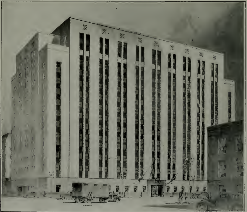
U. S. APPRAISERS STORES AND IMMIGRATION STATION UNDER CONSTRUCTION IN SAN FRANCISCO
