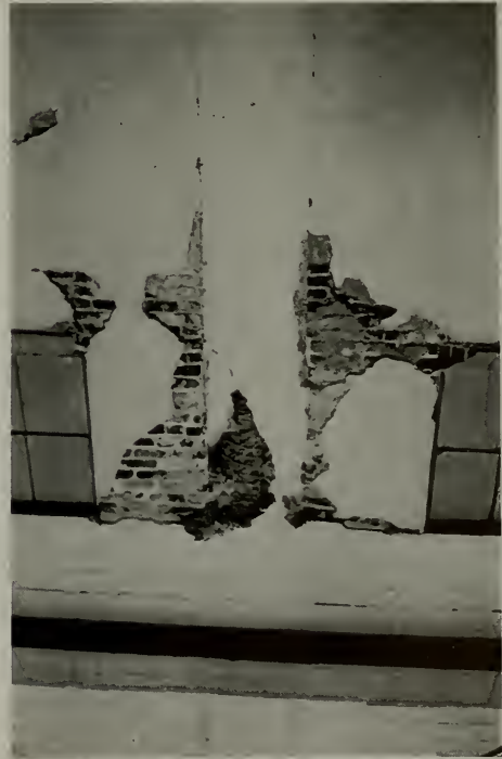
Looking northeast at Bekins Van & Storage Warehouse, Santa Barbara, California. Showing broken brickwork and possible cracked column.
