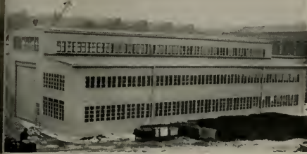
Apprentice building for the Harnischfeger Corporation
