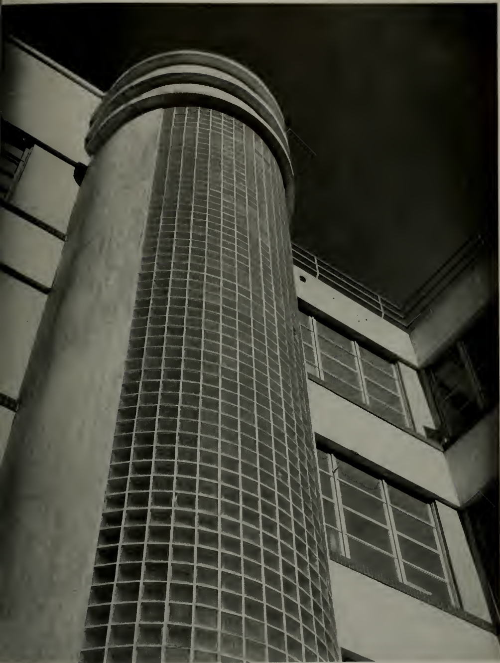
STAIR TOWER, SAMUEL GOMPERS TRADE SCHOOL, SAN FRANCISCO
