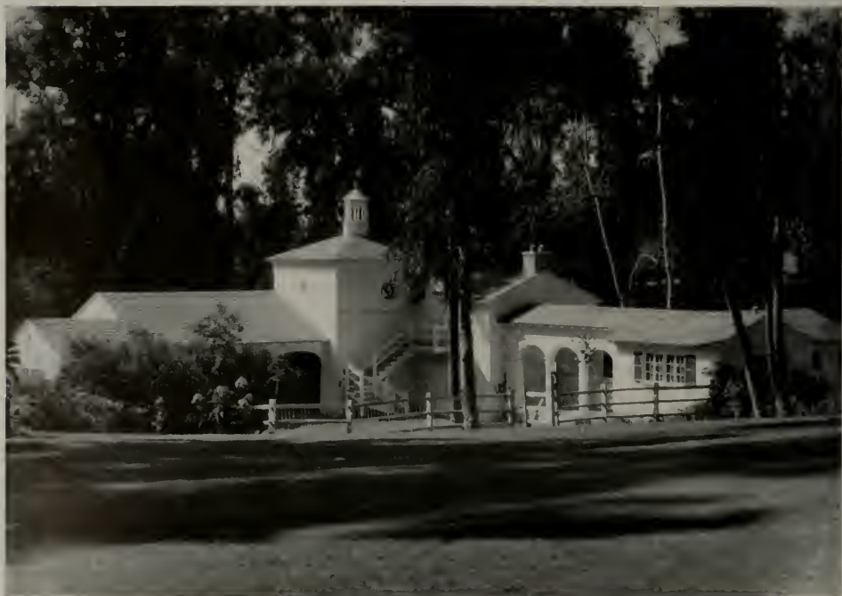
STABLES ON PRIVATE ESTATE, LOS ANGELES
