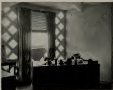
VIEW OF OFFICE SHOWING WALL TEXTURE
