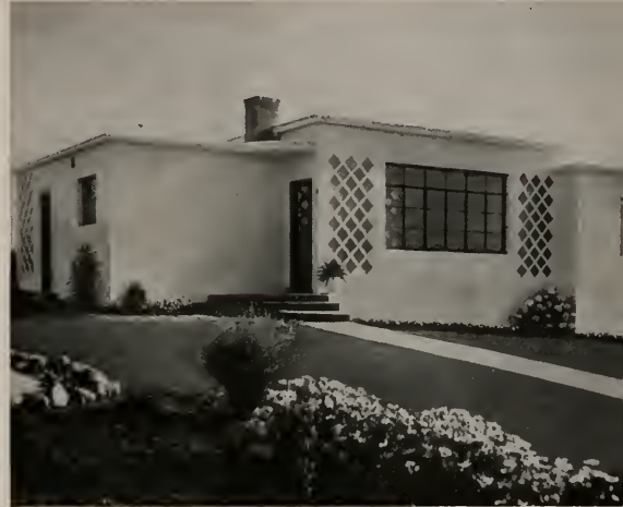
House completed; note pleasing architectural motif.
