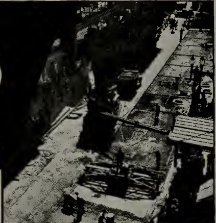
WED. Pouring concrete made with Golden Gate 24-Hour Cement on Post St. paving.
