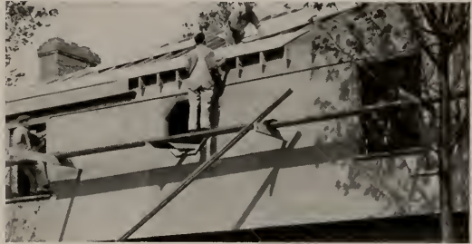
WALL SHEATHING The Plyscord-sheathed walls of this residence in Seattle, Wash., are 40% more rigid than if diagonal board sheathing had been used. The big panels also save up to 50% on sawing, fitting and joining... 50% on nailing. Tezays Francis Bellamy was the architect on this residence.
