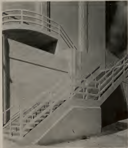
DETAIL OF BALCONY EXIT STAIRWAY
