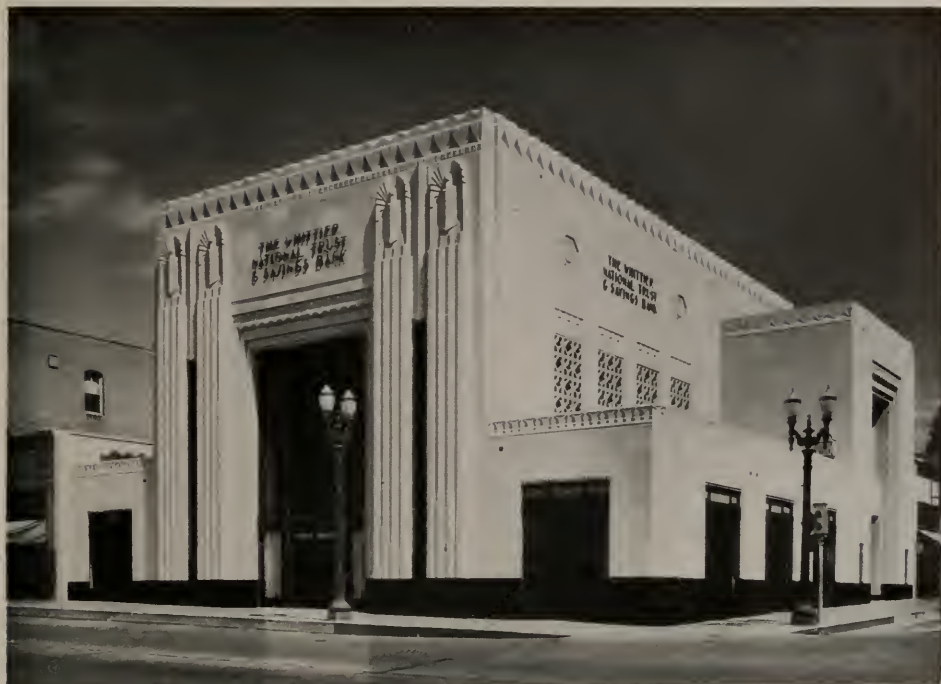
WHITTIER NATIONAL TRUST & SAVINGS BANK BUILDING, WHITTIER, CALIFORNIA William H. Harrison, Architect
