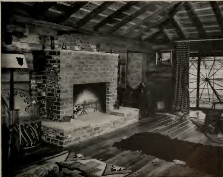
Fireplace below is built of red brick, suitable for ranch house or mountain lodge. Split bricks are spaced to allow a maximum of warm air passage.
