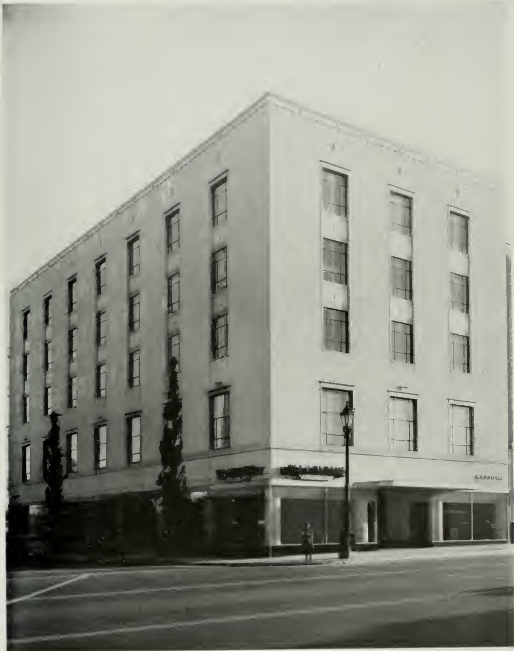
W. & J. SLOANE COMPANY, BEVERLY HILLS, CALIFORNIA JOHN PARKINSON AND DONALD B. PARKINSON, ARCHITECTS
