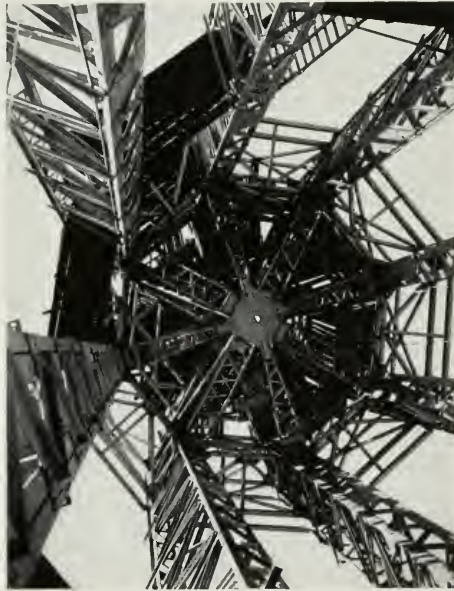
Detail of Tower Framework, Looking Up.
