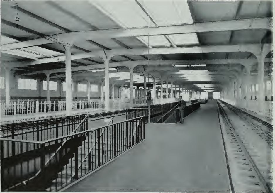
Bay Bridge electric railway trains enter and leave over this track level in the Terminal Building. Six tracks have been provided for Interurban (S. P.), Key System, and Sacramento Northern trains. Eleven ramps and fourteen stairways afford ample access to and from trains.
