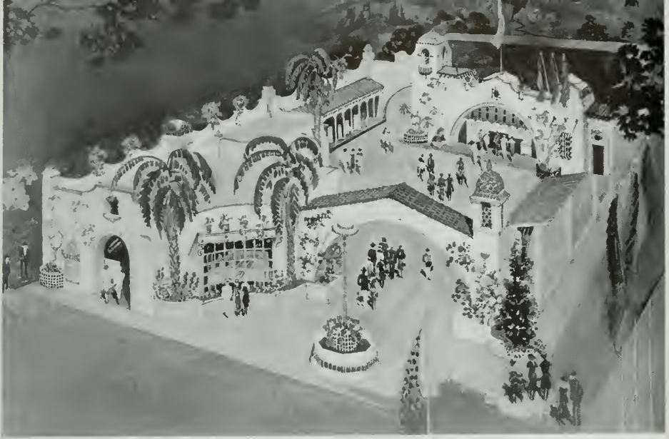
COOPERATIVE GAS INDUSTRY BUILDING AT TREASURE ISLAND
