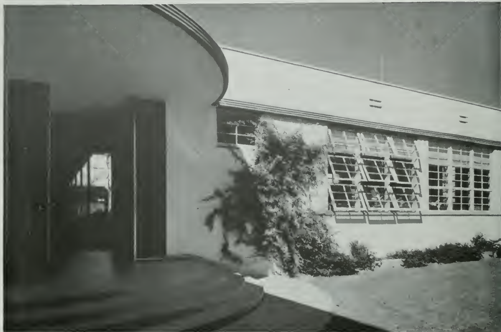
SOUTH PASADENA HIGH SCHOOL—ENTRANCE TO SCIENCE BUILDING
