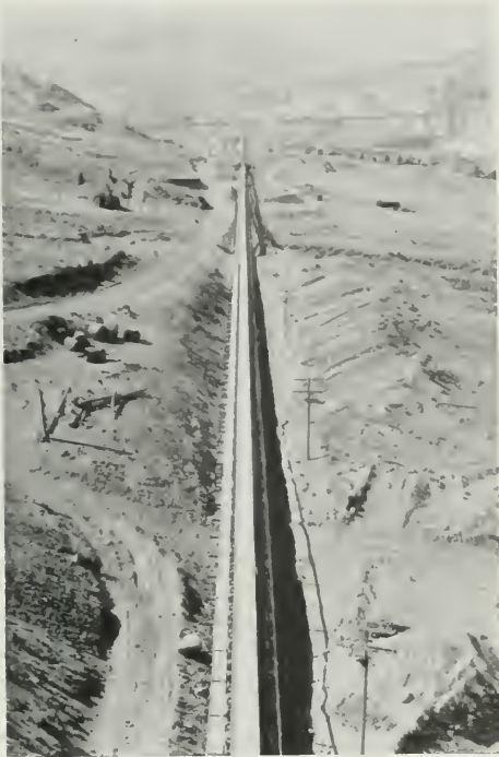
PICTURE SHOWS LENGTH OF WORLD'S LARGEST CONVEYOR BELT IN USE AT GRAND COULEE DAM, WASHINGTON STATE
