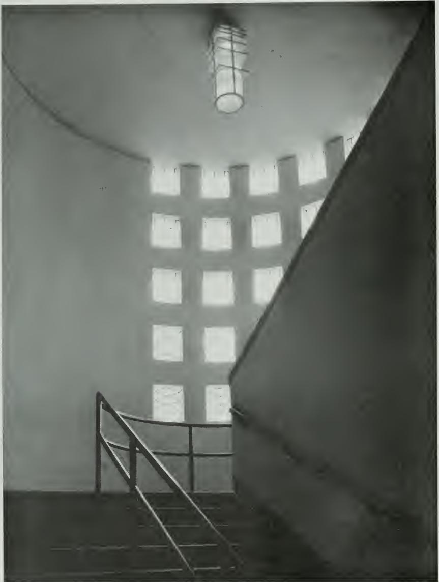
CONCRETE GRILLE WHICH LIGHTS THE MAIN STAIR HALL OF HOLLYWOOD HIGH SCHOOL MARSH, SMITH & POWELL, ARCHITECTS
