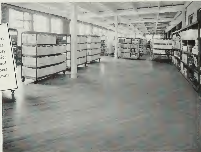
MFMA Northern Hard Maple floor in The Davidson Baking Company, Portland, Oregon
