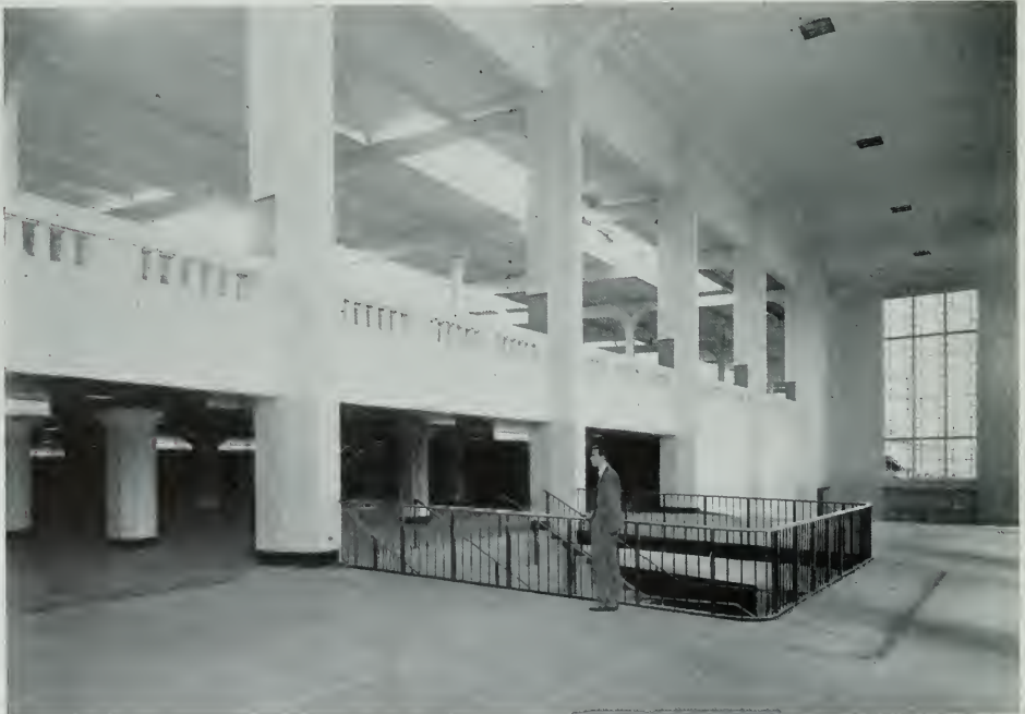
Passengers for Bay Bridge electric trains enter this foyer of the Terminal Building. The view, taken on the mezzanine floor, shows the track level to the upper left. Stairs in the center foreground lead to the street floor.
