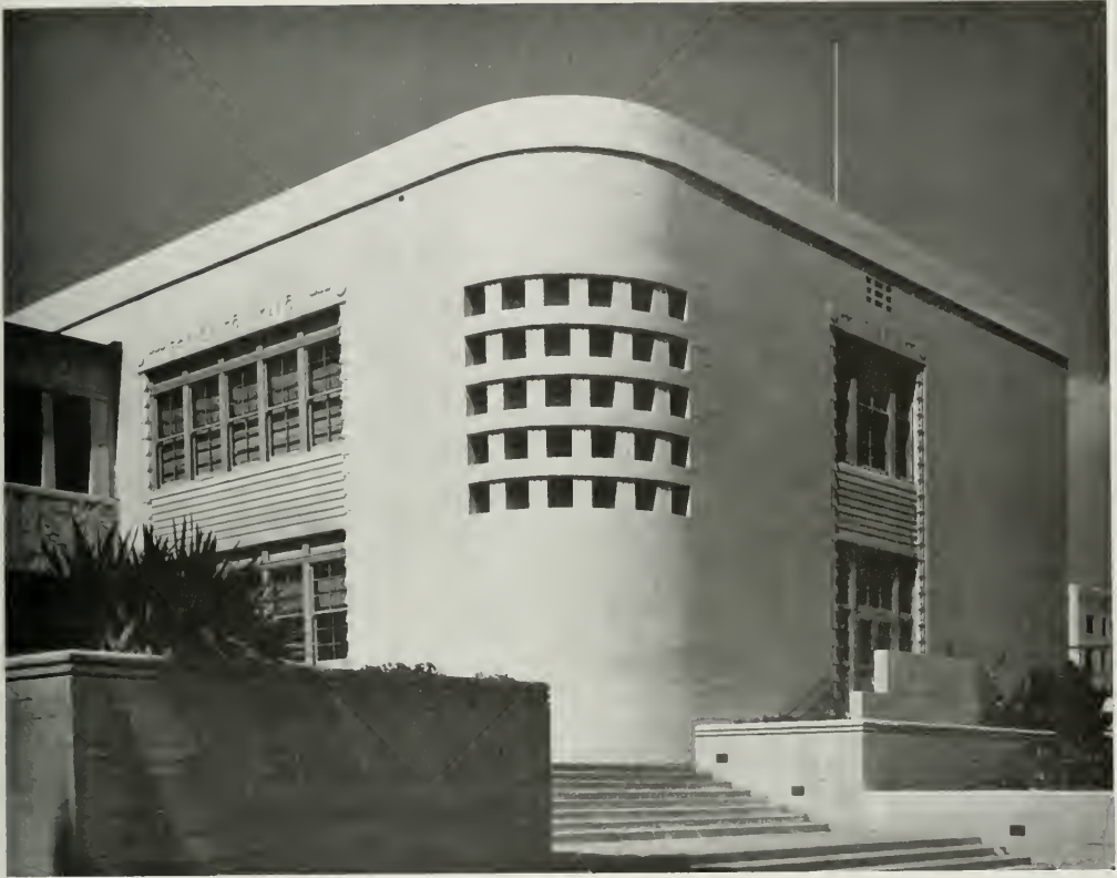
Millwork by Graves
