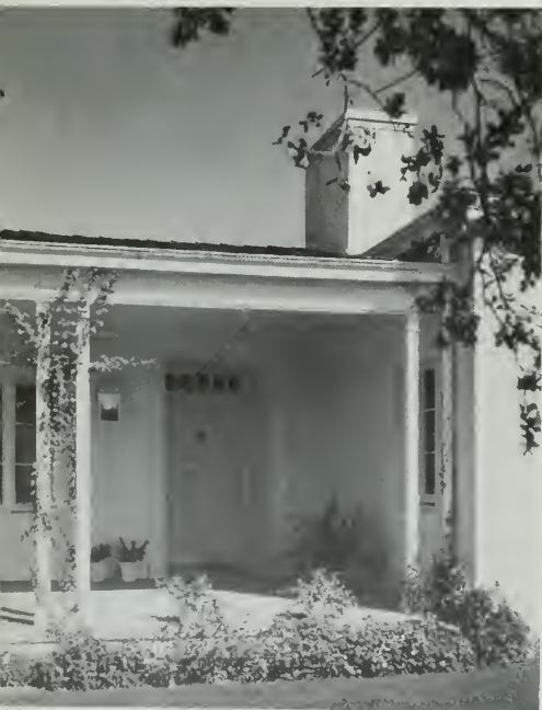
DETAIL OF ENTRANCE
