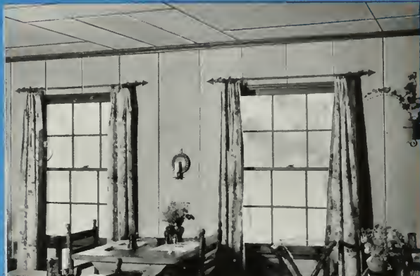
Infinite variety of pattern is possible with 5 standard sizes—16" x 16", 16" x 4', 16" x 8', 4' x 4', and 4' x 8'! Go up fast on open framing—jamb thickness—no cutting or sawing except at room borders and openings!
