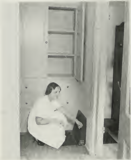
SAN GABRIEL VILLAGE DEVELOPMENT All units equipped with a Dual gas floor furnace
