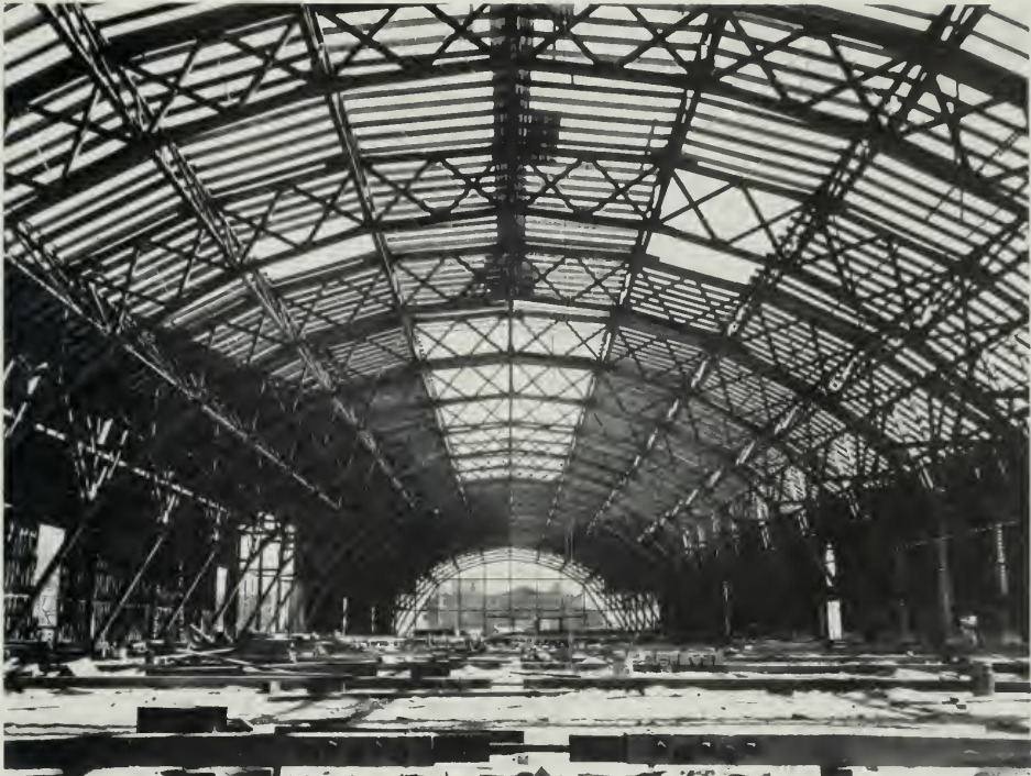
THREE-HINGED TIMBER ARCHES OF 200 FOOT SPAN, PREFABRICATED ROOF AND WALL PANELS, PALACE OF ELECTRICITY, GOLDEN GATE INTERNATIONAL EXPOSITION, TREASURE ISLAND
