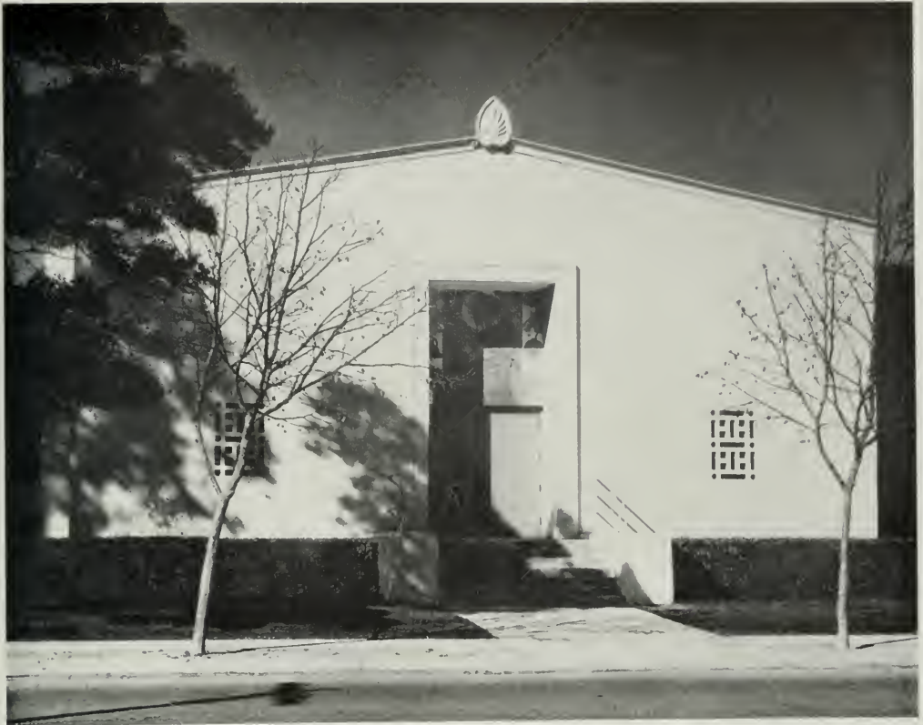
AUDITORIUM, HOOPER AVENUE SCHOOL, LOS ANGELES
