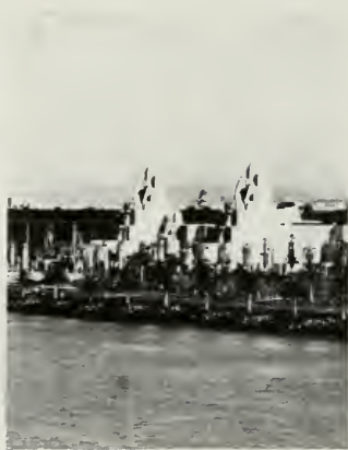
The Exposition is in effect a walled city, the western facades forming a barrier against the summer winds. The arriving visitor is embraced by the outstretched arms of entrance motifs. Variations of light and shade give colorful effect.
