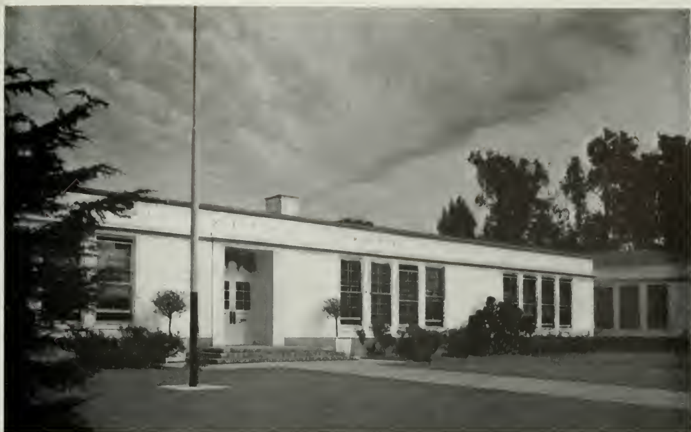
MILES AVENUE SCHOOL, HUNTINGTON PARK RALPH C. FLEWELLING, ARCHITECT
