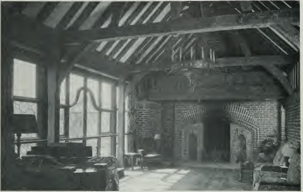
INTERIOR, LIVING ROOM, COTTAGE FOR OTIS R. MARSTON, BERKELEY
