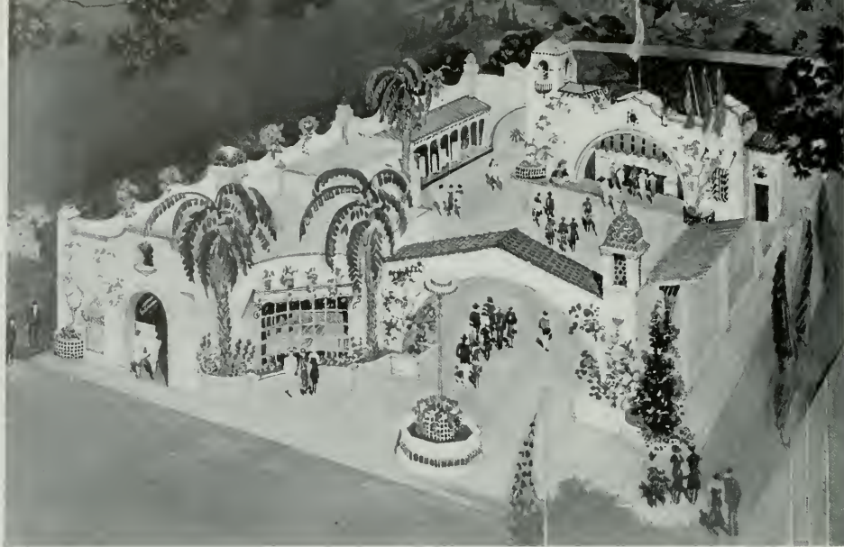
COOPERATIVE GAS INDUSTRY BUILDING AT TREASURE ISLAND
