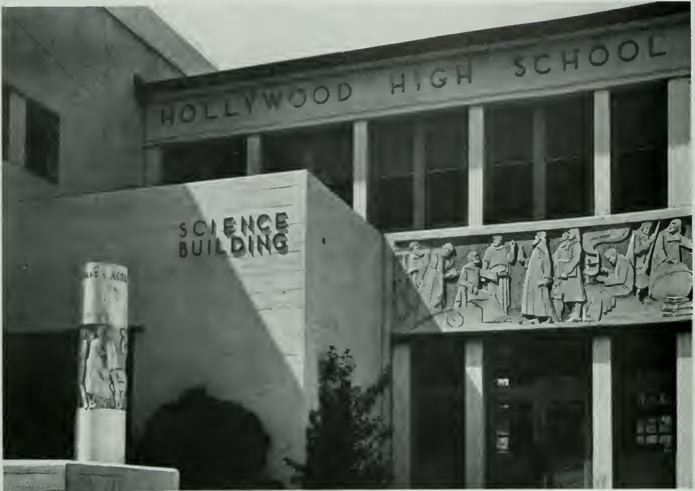
HOLLYWOOD HIGH SCHOOL, HOLLYWOOD, CALIFORNIA Marsh, Smith & Powell, Architects
