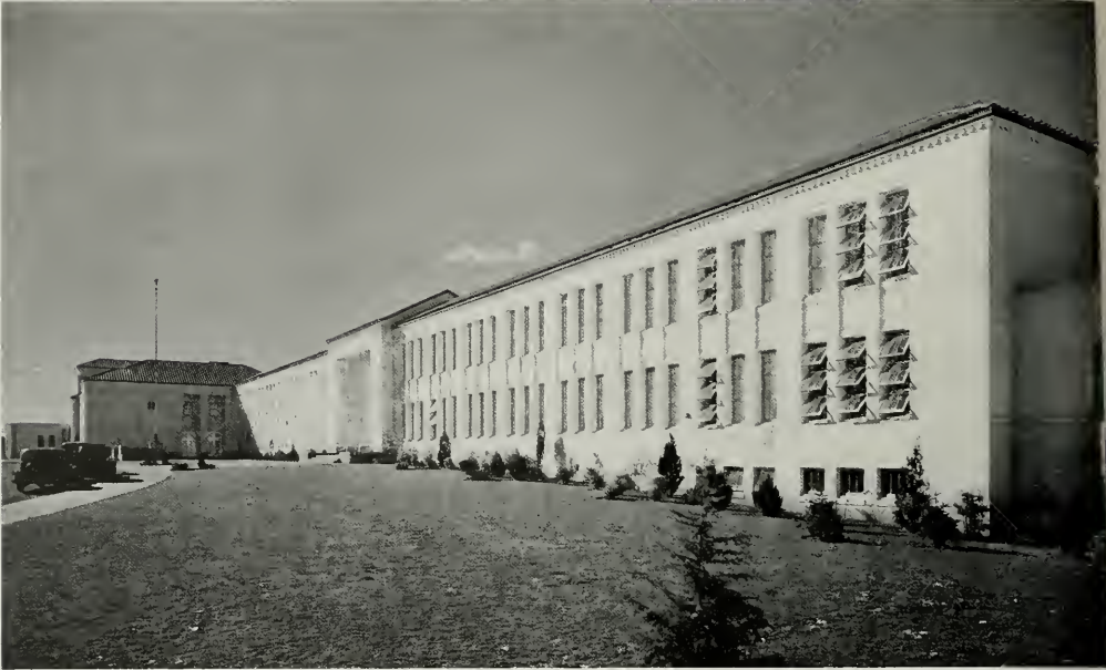
A CLASSIC SIMPLICITY CHARACTERIZES THE MAIN EASTERN FACADE, WELL SUITED TO THE CONCRETE CONSTRUCTION
