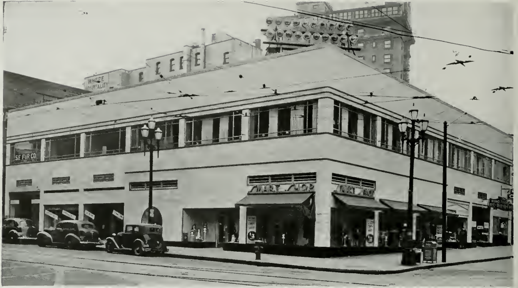
REMODELLED BUSINESS BUILDING, SEATTLE, WASHINGTON J. LISTER HOLMES, ARCHITECT
