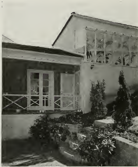
GARDEN VIEW, RESIDENCE OF MR. AND MRS. A. M. PILINSKY, OAKLAND, CALIFORNIA Earl R. MacDonald, Architect
