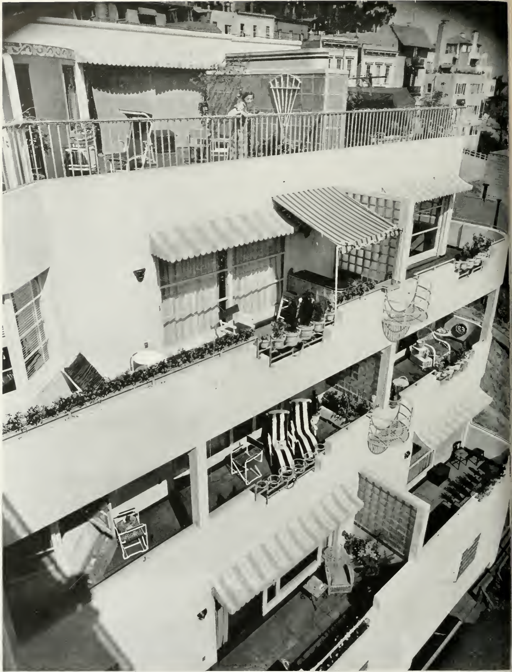
REAR ELEVATION OF APARTMENT HOUSE AT 1360 MONTGOMERY STREET, SAN FRANCISCO, SHOWING UNIQUE STEP-BACK ARRANGEMENT WHICH PROVIDES UNUSUAL OUTDOOR COMFORT
