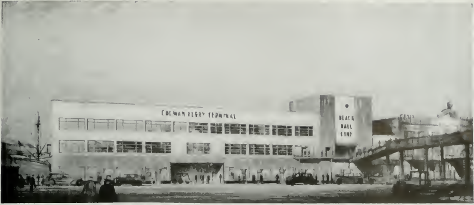
COLMAN FERRY TERMINAL, SEATTLE, WASHINGTON ARTHUR L. LOVELESS AND LESTER FEY, ARCHITECTS
