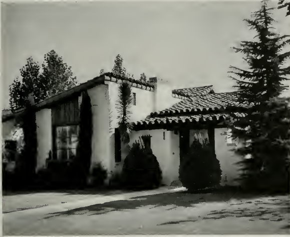
Residence of J. W. Hall, Fresno, California
