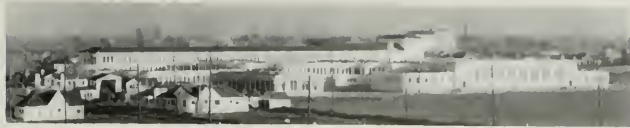
The suggestion of a great industrial plant is particularly striking in this view from athletic grounds on the west.
