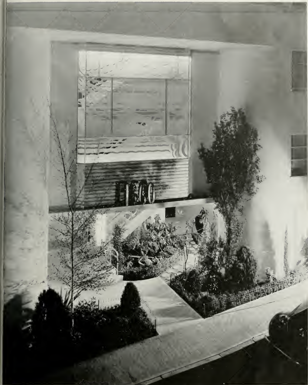
MAIN ENTRANCE OF APARTMENT HOUSE AT 1360 MONTGOMERY STREET, SAN FRANCISCO, SHOWING CLOSE UP OF SANDBLASTED GLASS PANEL, ILLUMINATED AT NIGHT BY CONCEALED LIGHTS
