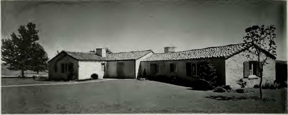
RESIDENCE OF J. J. ECTOR, YAKIMA WILLIAM J. BAIN, ARCHITECT
