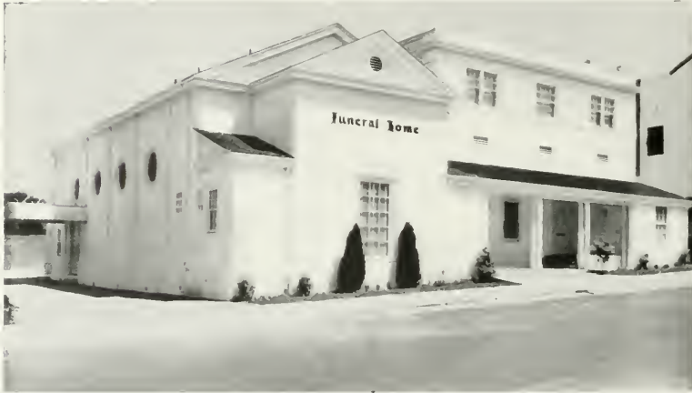
FUNERAL HOME AFTER ALTERATIONS Frederick H. Reimers, Architect
