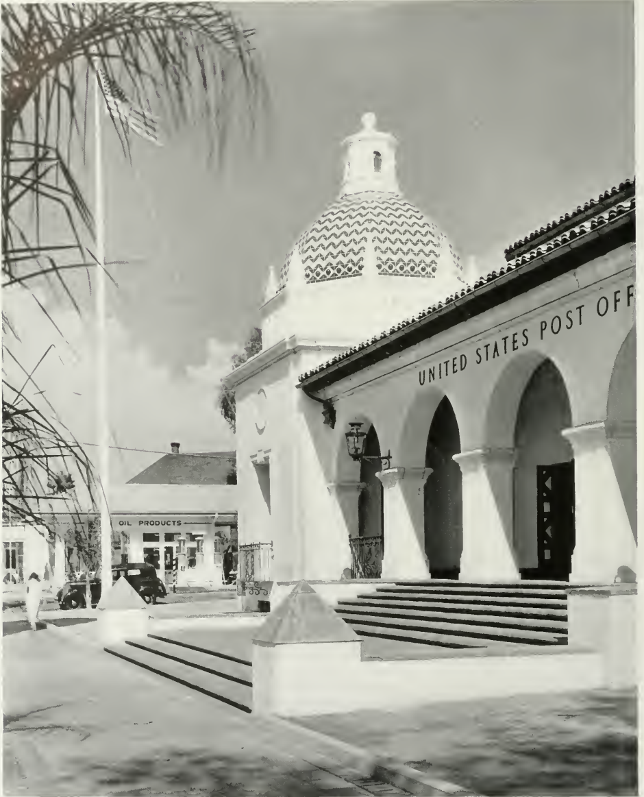
THE DOME, POST OFFICE, REDLANDS, CALIFORNIA G. STANLEY WILSON, A. I. A., ARCHITECT
