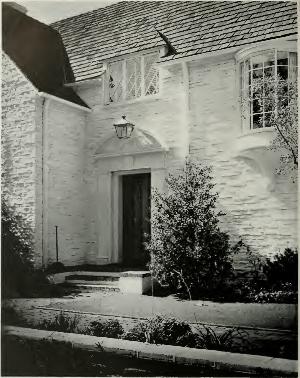
ENTRANCE DETAIL, CONCRETE MASONRY RESIDENCE OF MR. AND MRS R. J. PRINGLE BEL-AIR, CALIFORNIA H. ROY KELLEY, ARCHITECT
