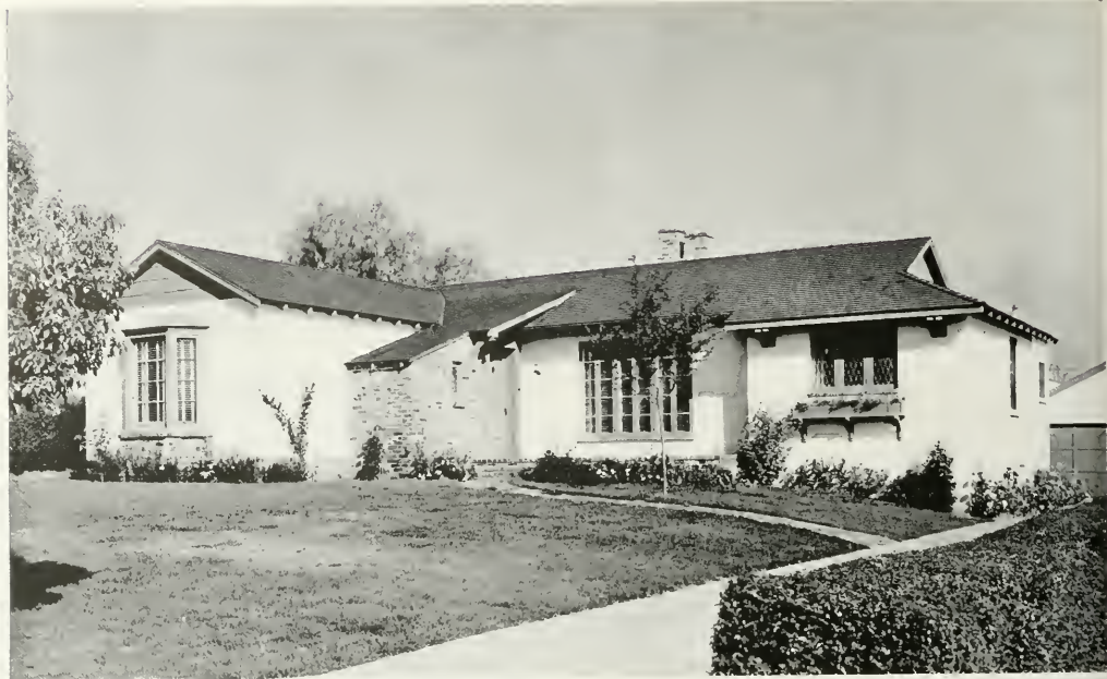
HOME OF MR. AND MRS. KENNETH WEISER, GLENDALE, CALIFORNIA ERWOOD P. EIDEN, ARCHITECT
