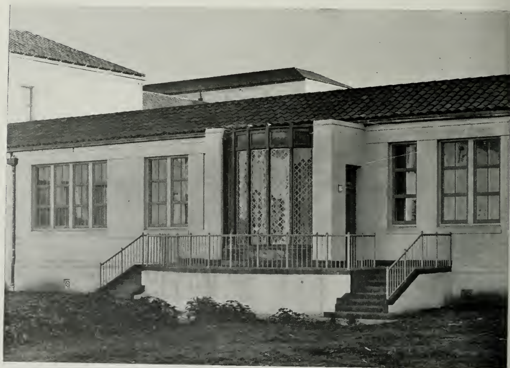
THE DOMESTIC SCIENCE DINING ROOM BAY OVERLOOKS THE FOUNTAIN COURT
