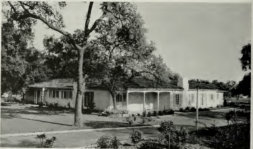
ANOTHER VIEW, REINFORCED CONCRETE HOUSE OF JOHN D. GREGG, ARCADIA GARRETT VAN PELT, ARCHITECT
